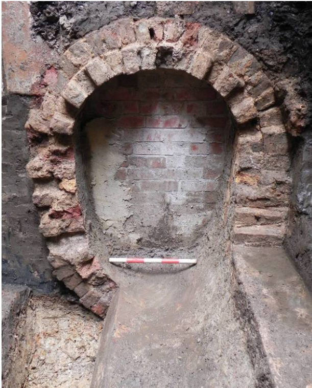
Photo 7: Profile of sewer [535], backfilled and bricked up westward, and largely broken out within the trench (looking west).
