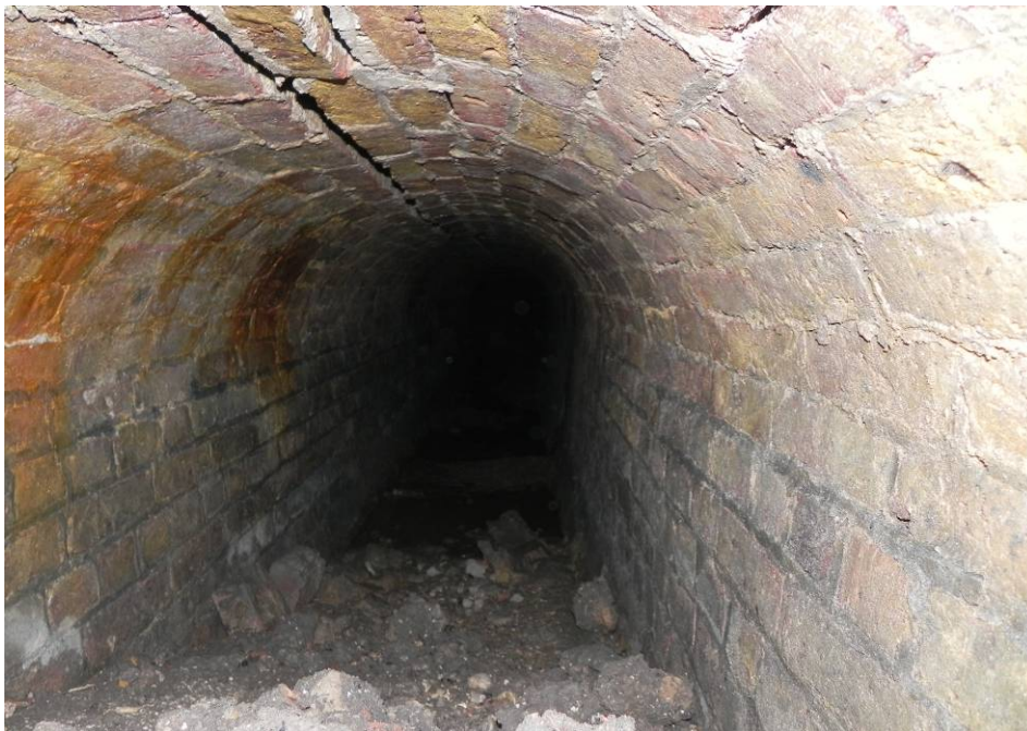
Photo 10: Trench 2 – Interior of Victorian brick sewer [535] (looking east).
