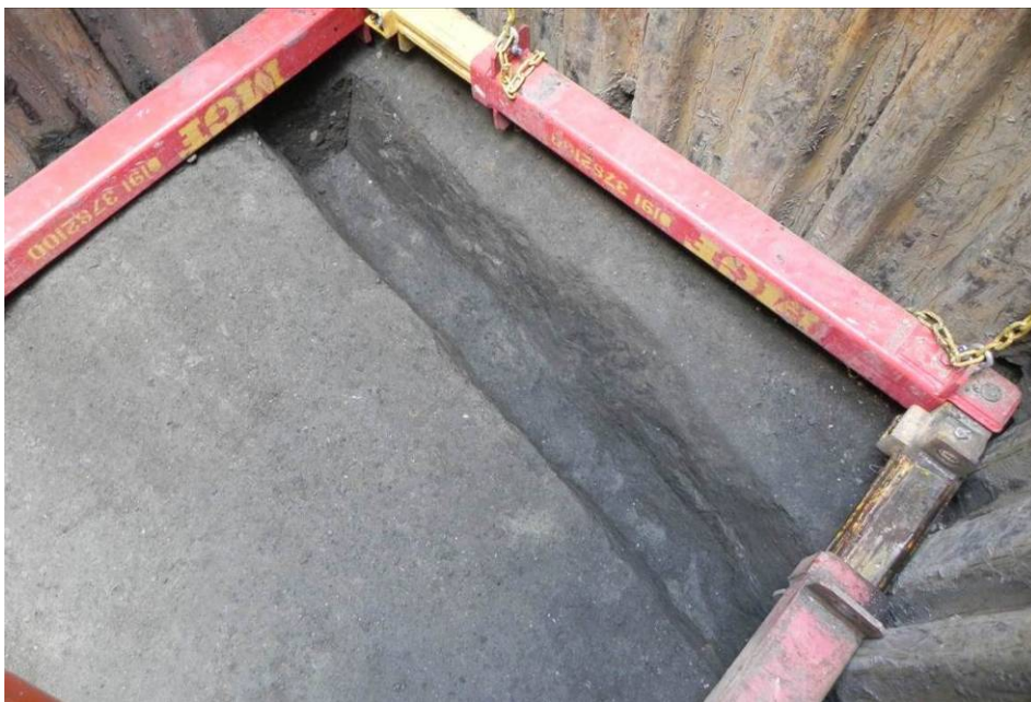
Photo 18: Trench 13 – Beam slot [302] (looking south-east).
