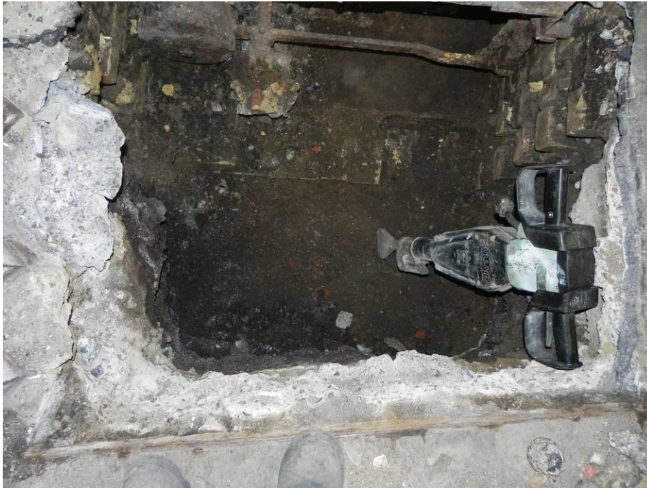
Photo 19: Railway Tavern Trial Pit- Foundations of the Railway Tavern with 19th-century walls, disused machinery, and construction backfill (north at top)
