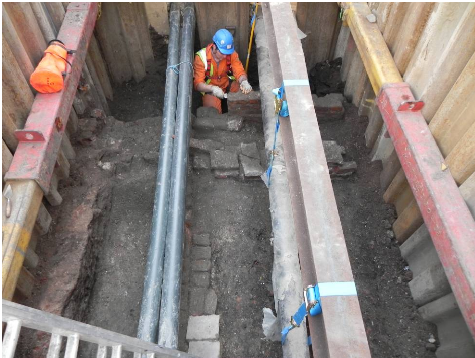
Photo 4: Trench 1 – Post-medieval brick structures, including wall [325] (left), drain [321] (centre to centre right), wall [332] (top), floor [329] (centre bottom) (looking east).
