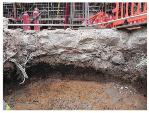
Photo 1 Trench 4 looking North. Section showing gravelly brickearth natural overlain by clay and marsh deposits.
