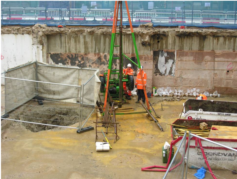
Photo 3 Borehole 1. Looking east. During drilling
