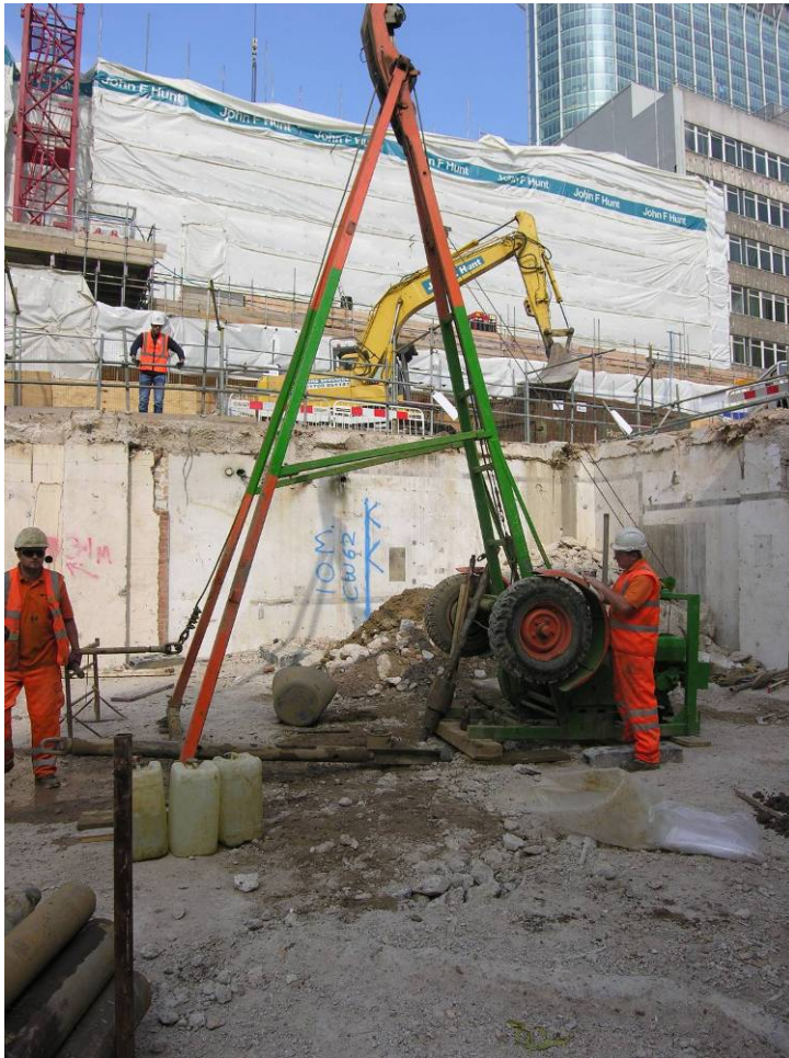
Photo 4 Looking north-west. Borehole 3 during drilling
