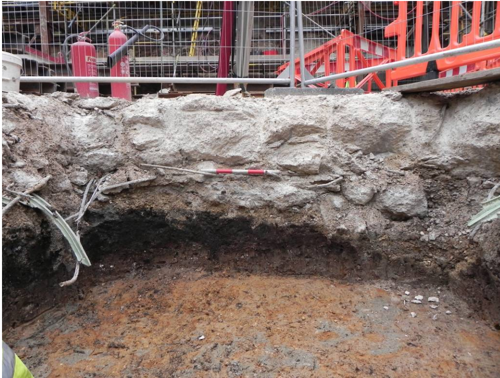
Photo 1 Trench 4 looking north. Section showing gravelly brickearth natural overlain by marsh deposits.
