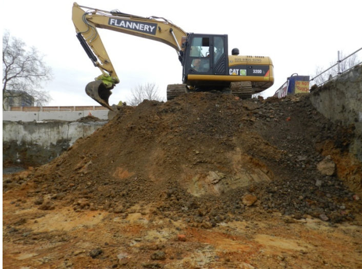
Photo 14 bulk excavation of south area of shaft
