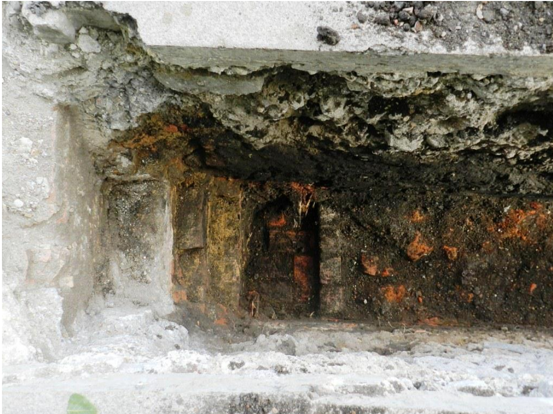
Photo 19 Culvert [336] (north is top) East trench
