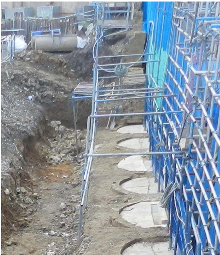
Photo 4, Rail Wall [21] during demolition
