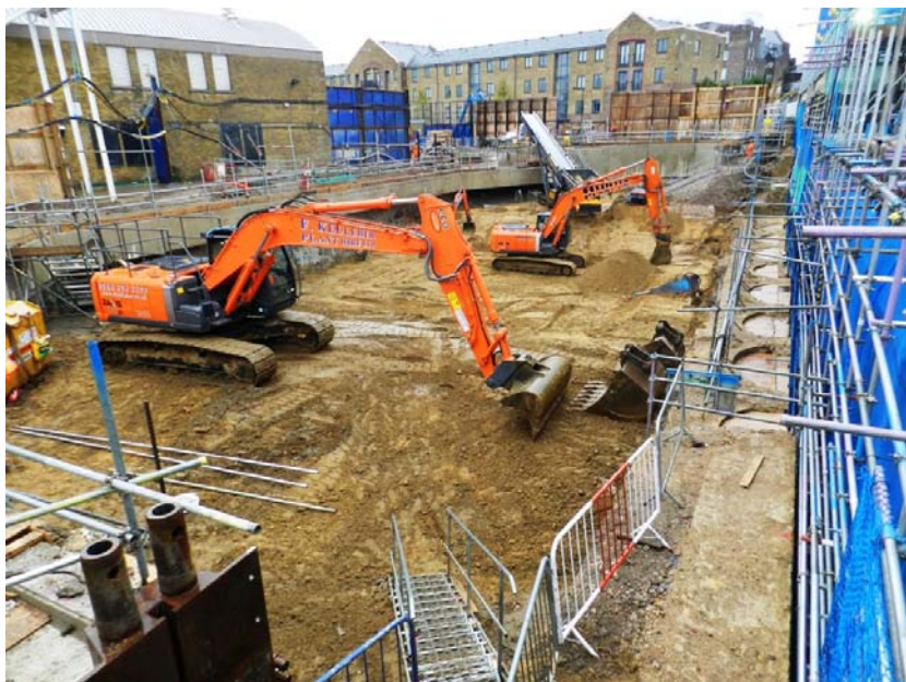
Photo 1, General ground reduction and removal of rail wall
