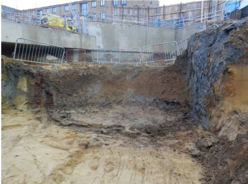
Photo 3, Section through “tank” [17]
