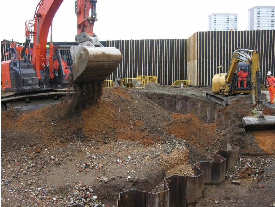
Photo 2, General ground reduction of modern overburden in the Ventilation Shaft
