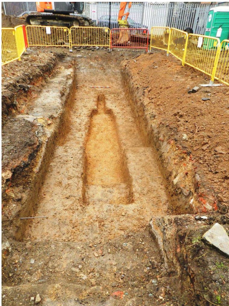
Photo 1, Temporary Access Shaft Evaluation Trench, showing reworked brickearth [2], and the slot dug to expose the natural terrace gravels [1], looking north
