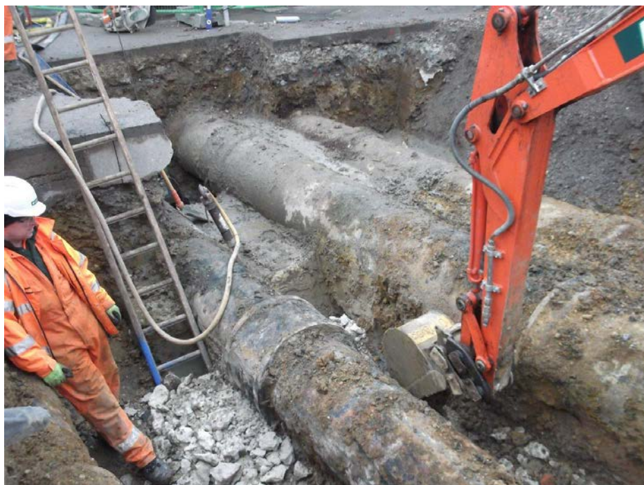
Photo 2 Excavating between pipes at 103.5m ATD (approx.)
