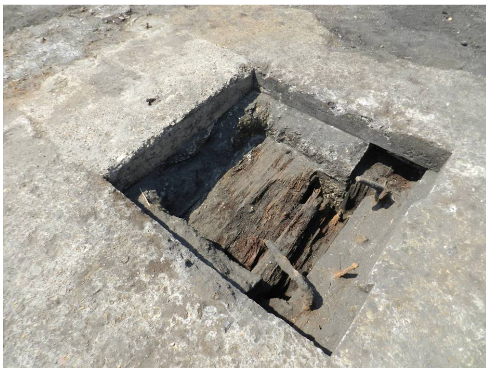
Photo 6 Concrete and timber structure [104/114] A possible hoist or crane base. (Looking north)
