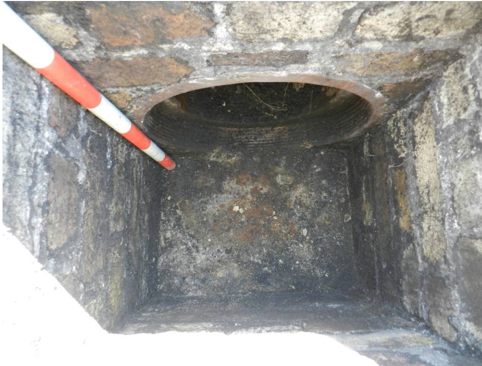
Photo 7 Drain [111]. (South-west at top of picture).
