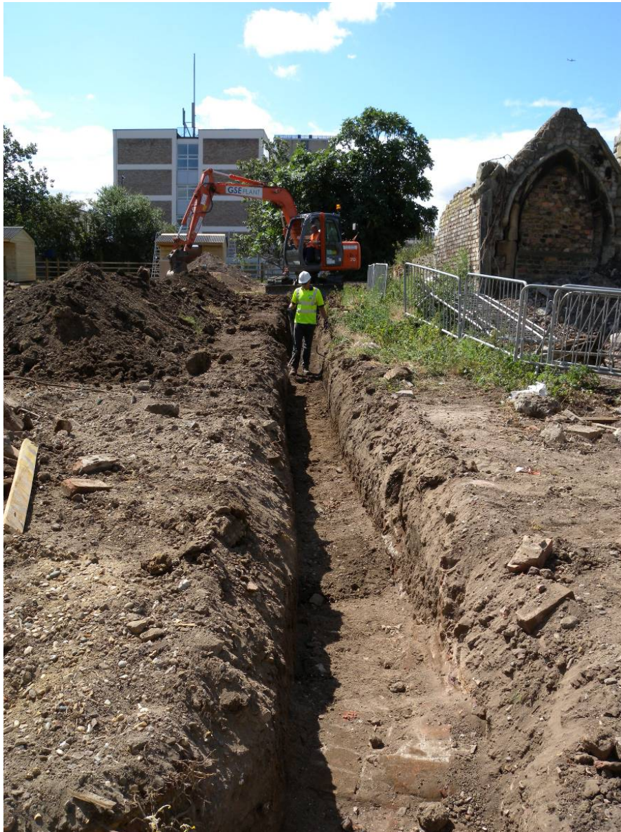
Water pipe trench, looking south, with 20th-century walls (front)
