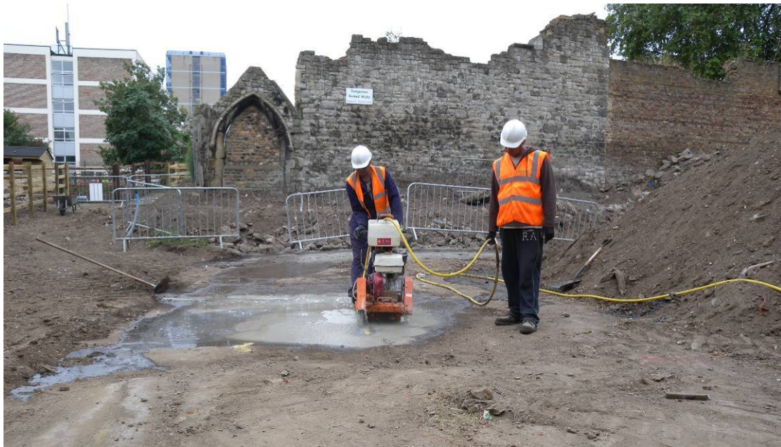
Cutting concrete, Stepney City Farm, looking south
