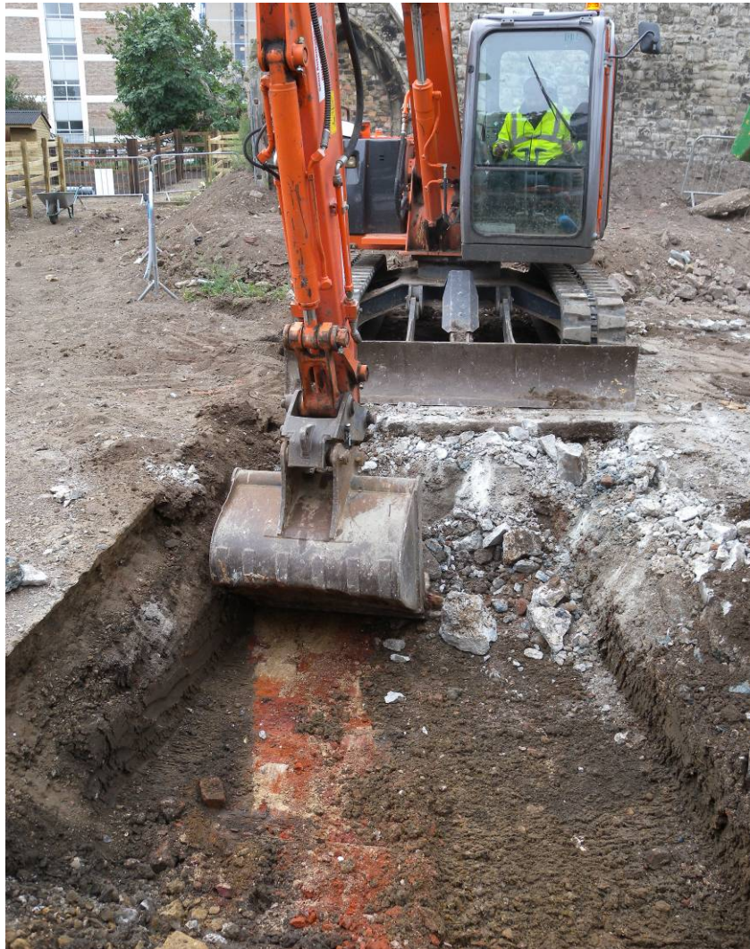
Machine excavating ground for a pig wallow, 20th-century brick wall (centre).
