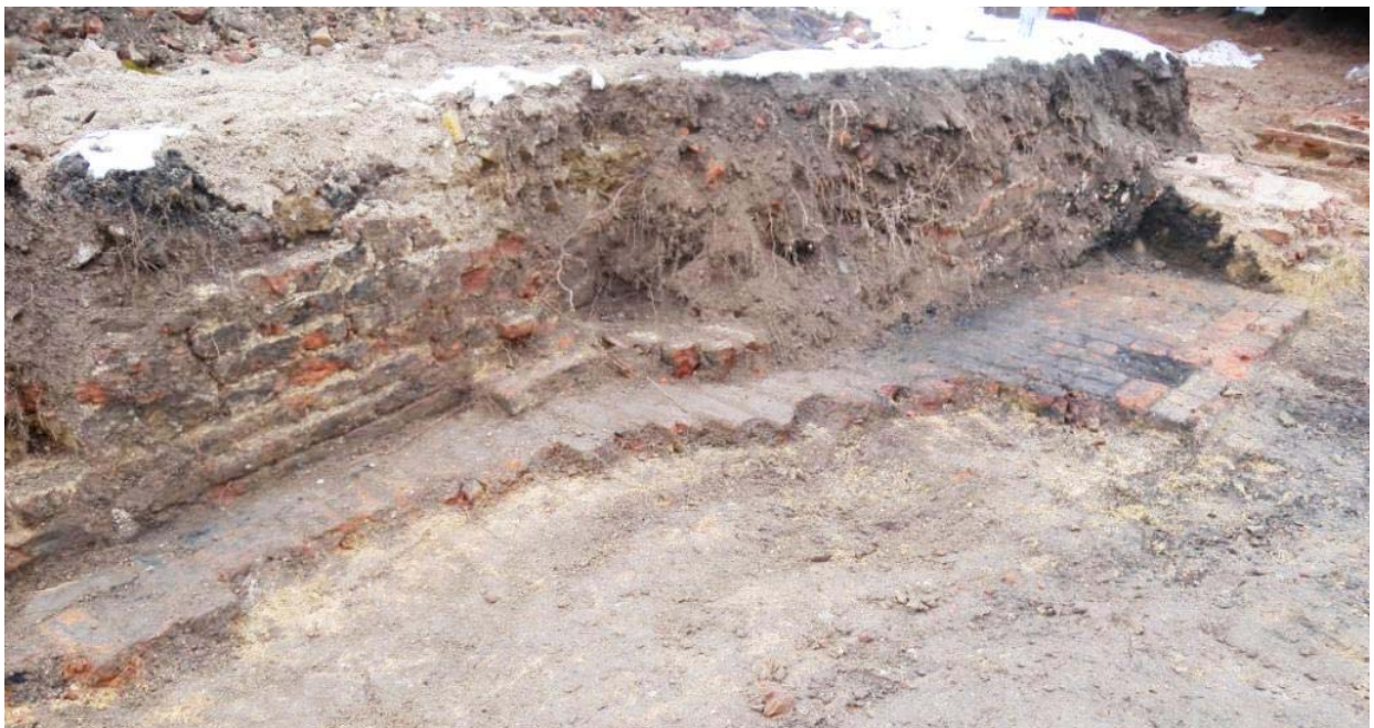
Coal cellar north end of Trench 2, built over part of the massive foundations exposed in Trench 1
