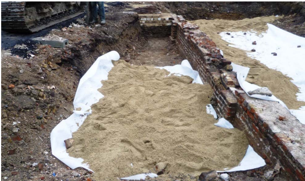
Photo 22 Geotextile and sand in trench 3
