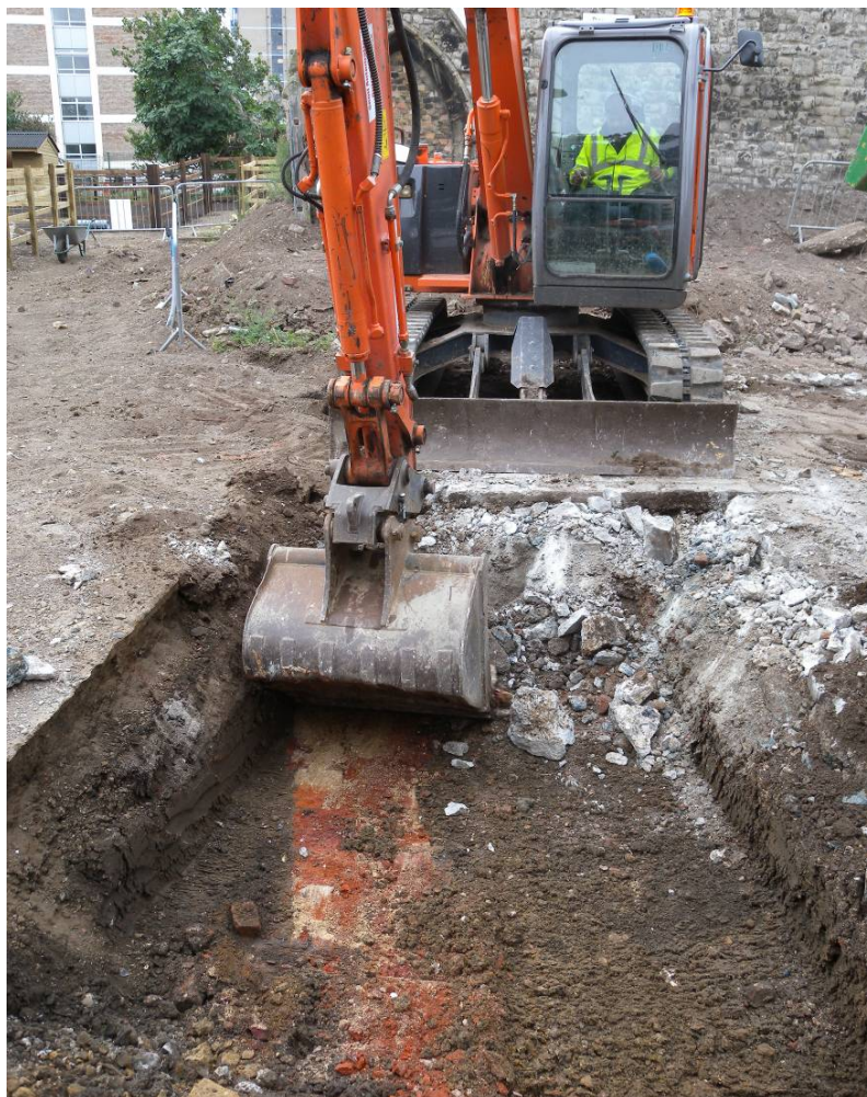
Photo 4 Machine excavating ground for a pig wallow, 20th-century brick wall (centre).
