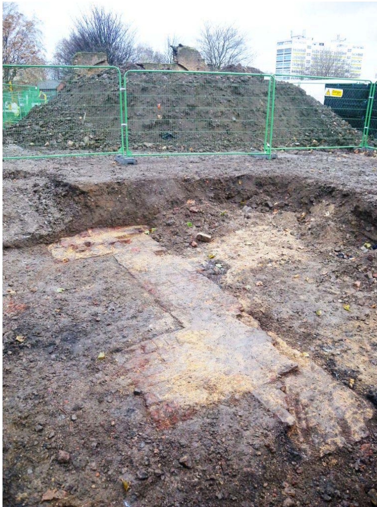
Photo 19 Foundations of the Congregational church
