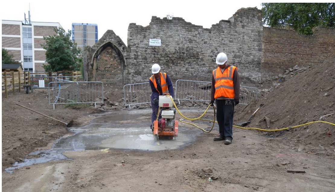
Photo 3 Cutting concrete, Stepney City Farm, looking south
