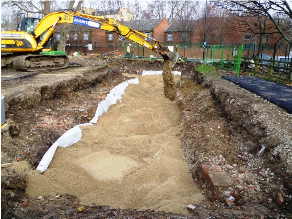
Photo 23 Sand filling trench 3 to 200mm above brick remains at side of trench
