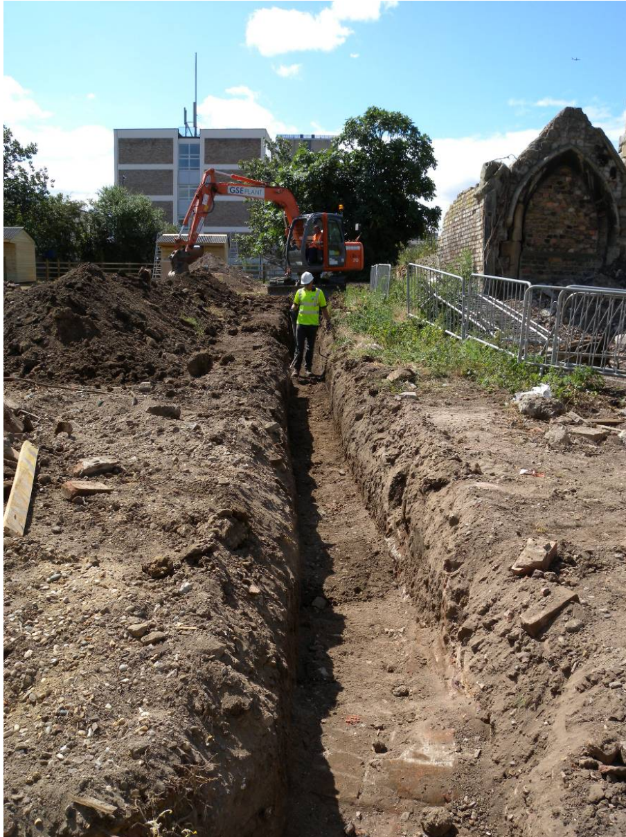
Photo 1 Water pipe trench, looking south, with 20th-century walls (front)
