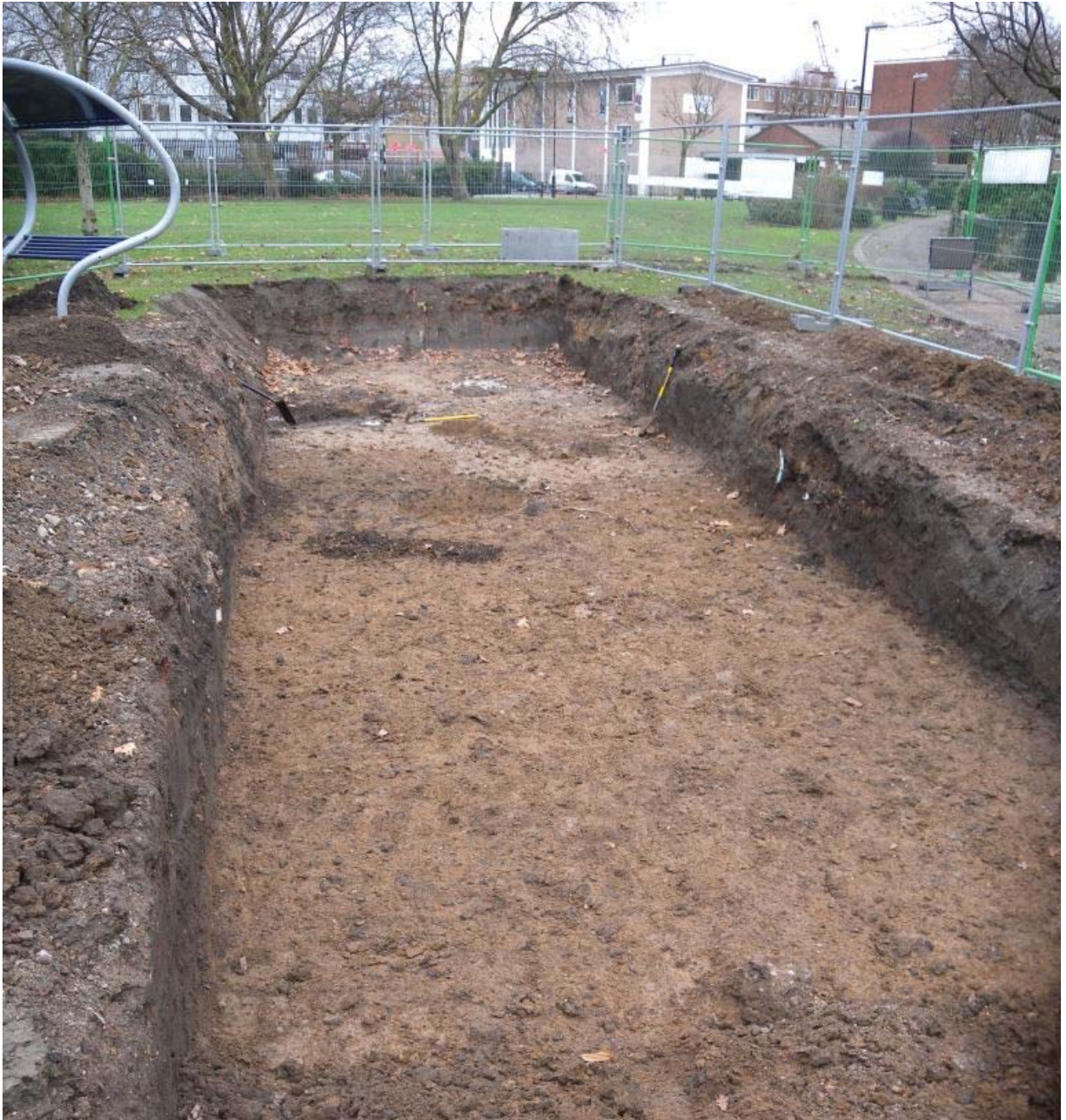
Photo 16 Trench 6, looking south
