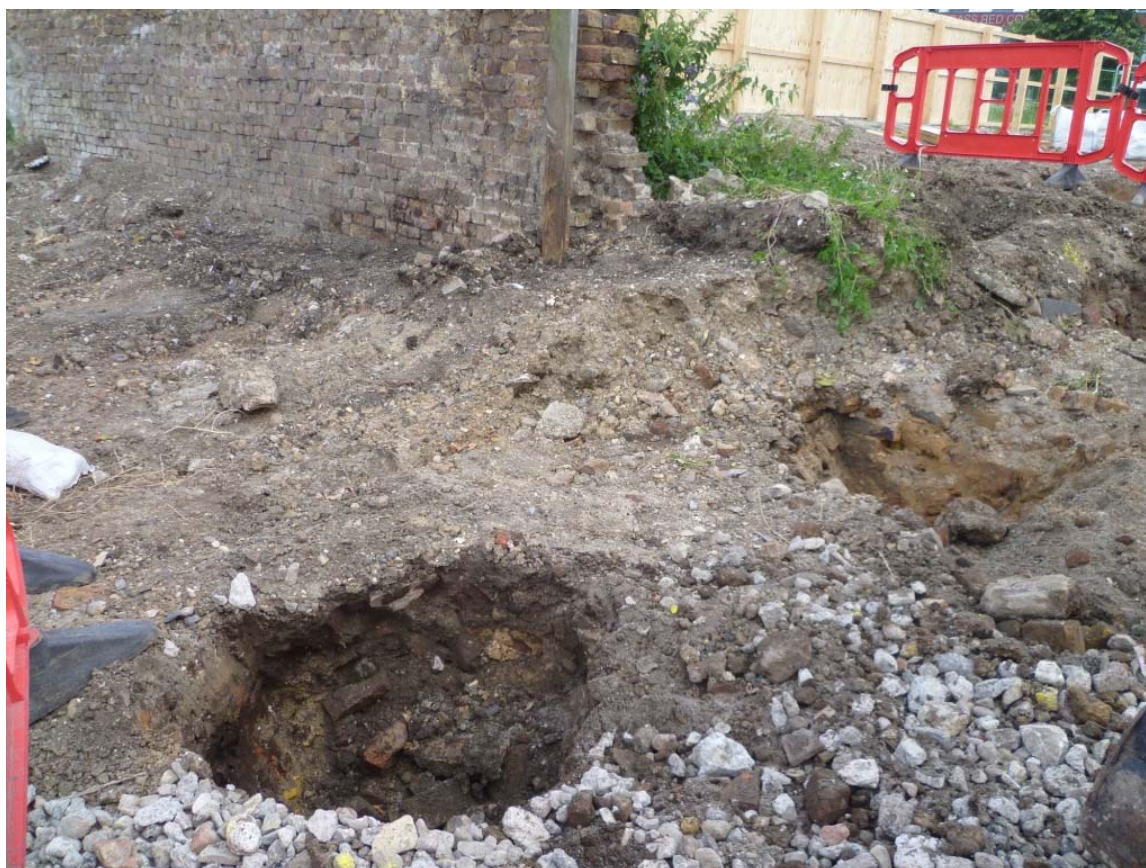
Photo 13: Fence post holes around west edge of church wall, looking south-east
