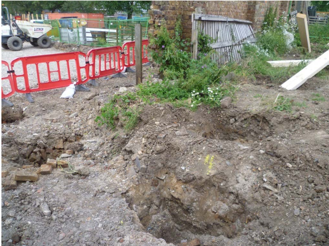
Photo 12: Fence post holes south of Church Wall, looking north-east
