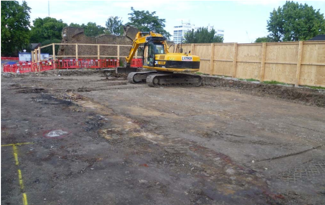
Photo 7: Ground reduction exposing the top of Congregational Church wall foundations, south of the freestanding section of Congregational Church
