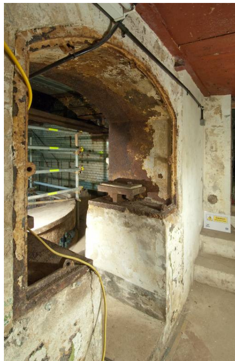
Fig 14 The access to the basement room containing the well (08512036)
