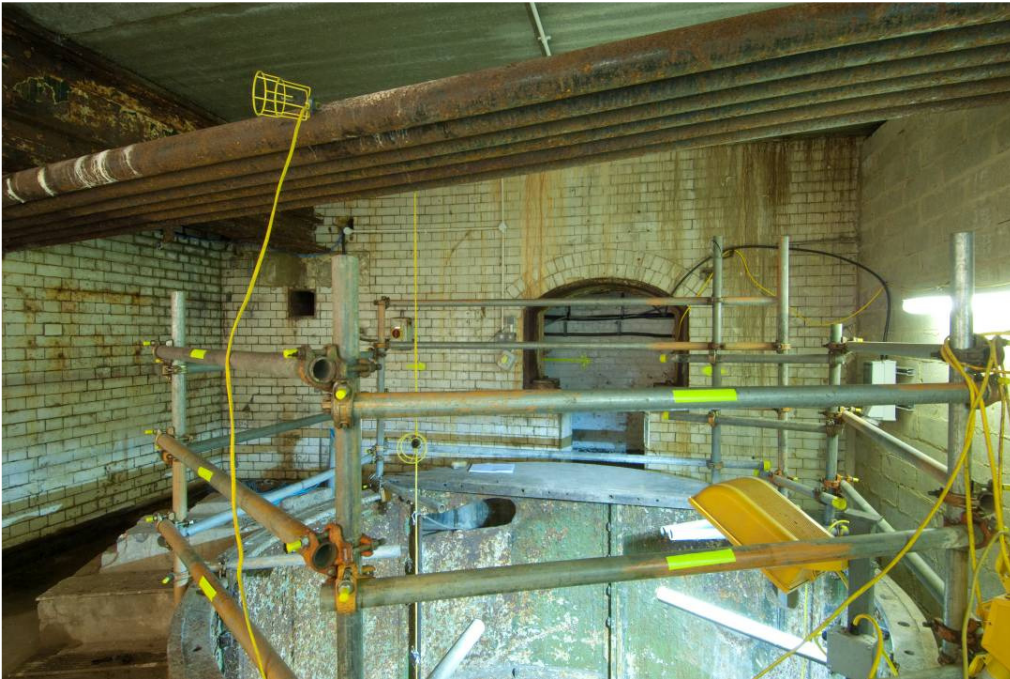
Fig 7 View of the basement room containing the well, looking south (08512001)
