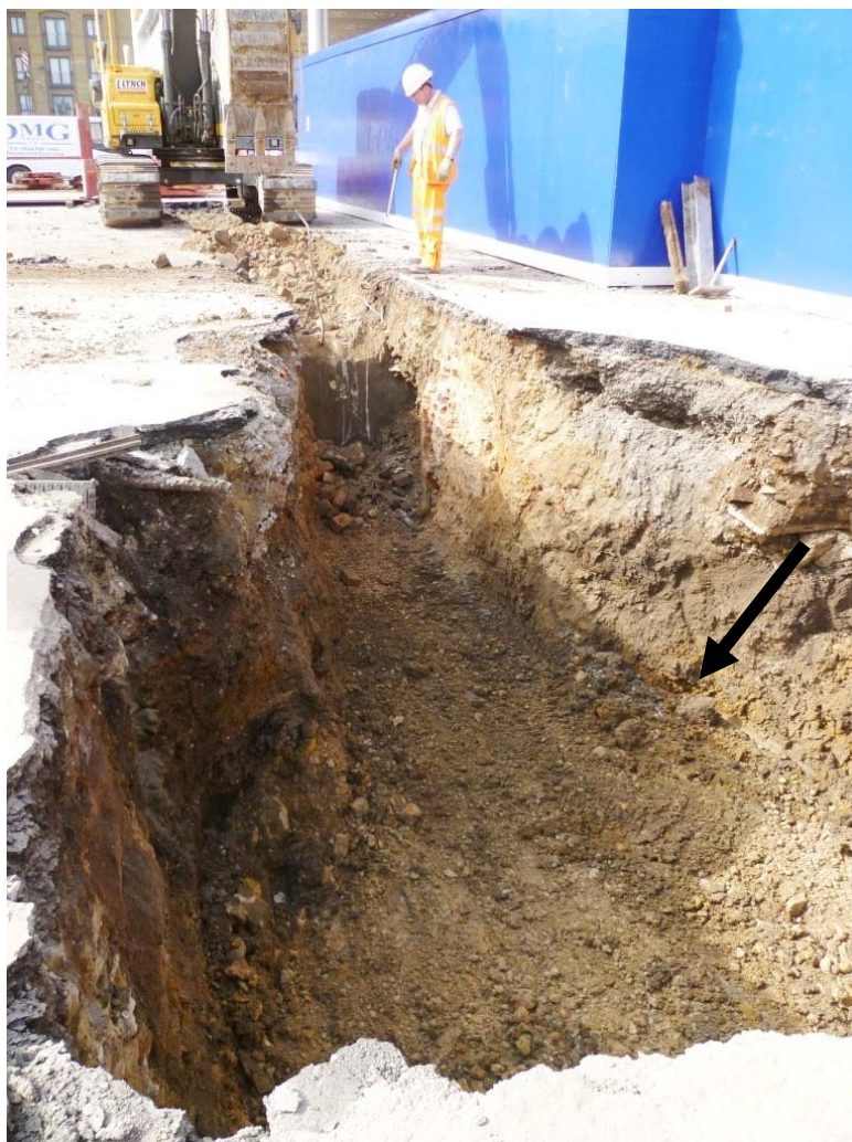
Photo 6: Eastern Manhole and Drainage trench: Looking west, showing Albion Brewery brick and concrete foundations cutting through archaeologically sterile natural deposits with a blackish waterlain silt (arrowed), cut through by Albion Brewery basements in the distance
