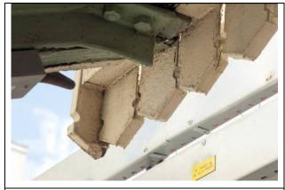
Fig 15 Detail of the dentelled wooden edging on former Platform 2
