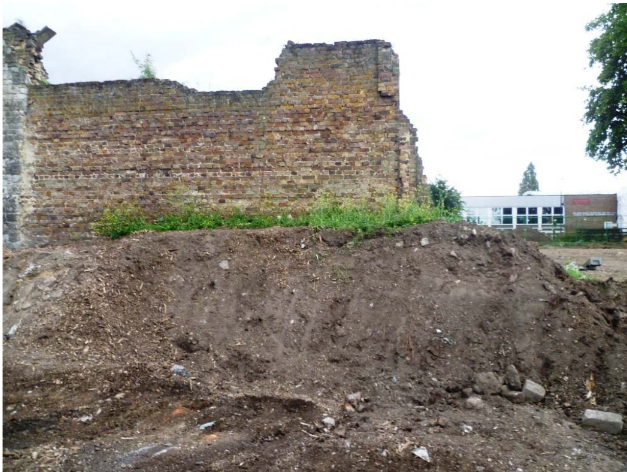
Photo 7 Removal of first metre of modern fill
