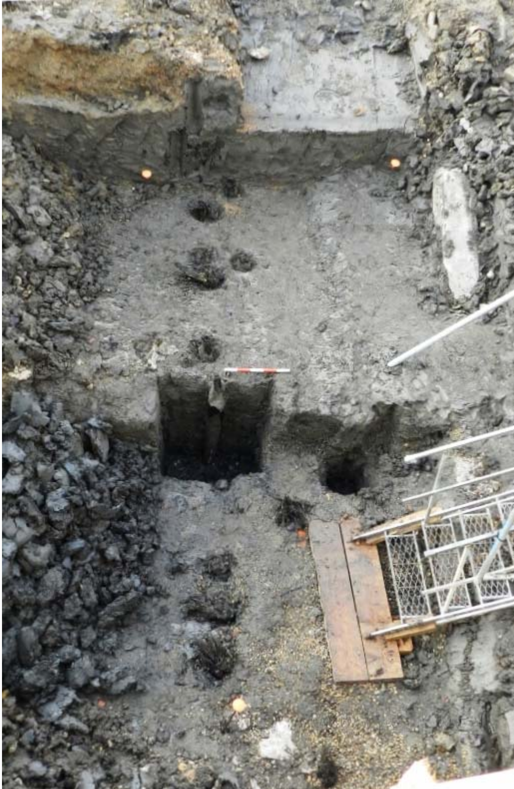
Photo 2 Oblique overview of timber structure, 23rd November 2011, looking north-west
