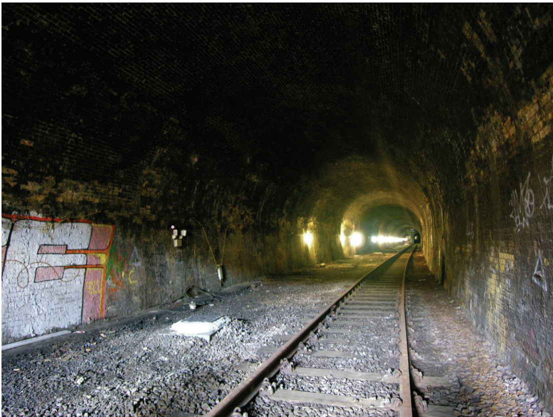
Fig 5 General view of the tunnel interior, looking north.
