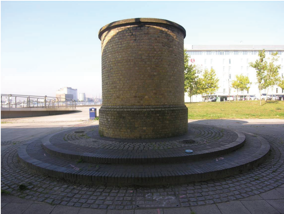
Fig 10 Northern tunnel vent superstructure, looking west.
