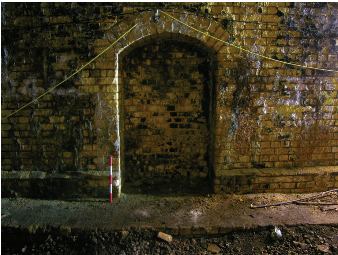
Fig 9 Tunnel refuge, looking east
