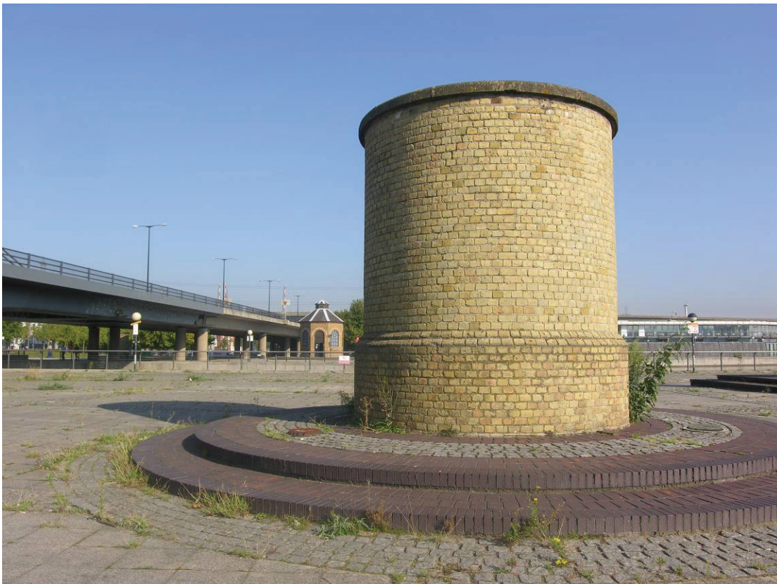
Fig 11 Southern tunnel vent superstructure with pump house in the background, looking north.
