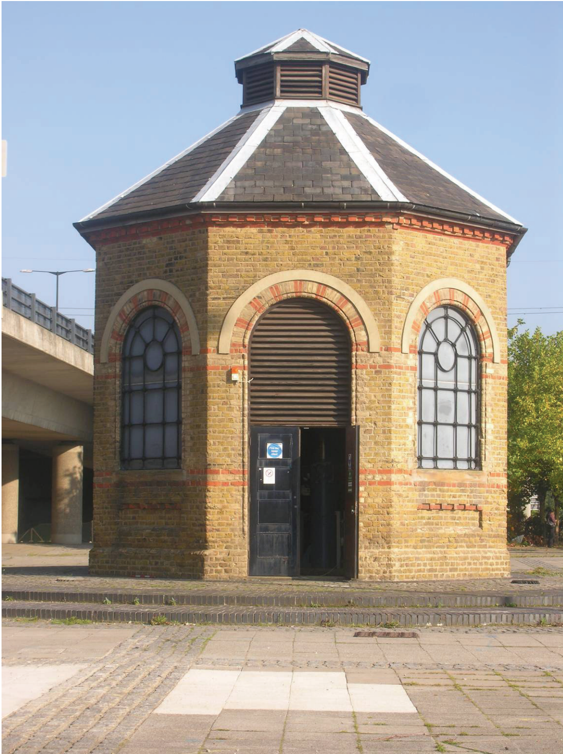
Fig 12 View of the pump house built at the same time as the tunnel in order to pump out water which leaked in from the Albert Dock above, looking north.
