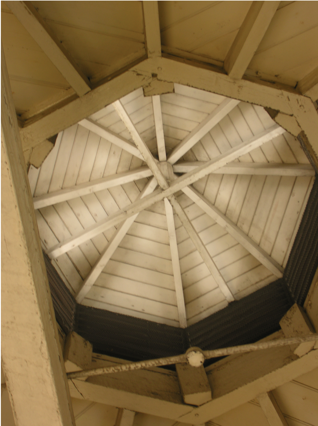
Fig 14 Interior view of the timber roof structure of the pump house.
