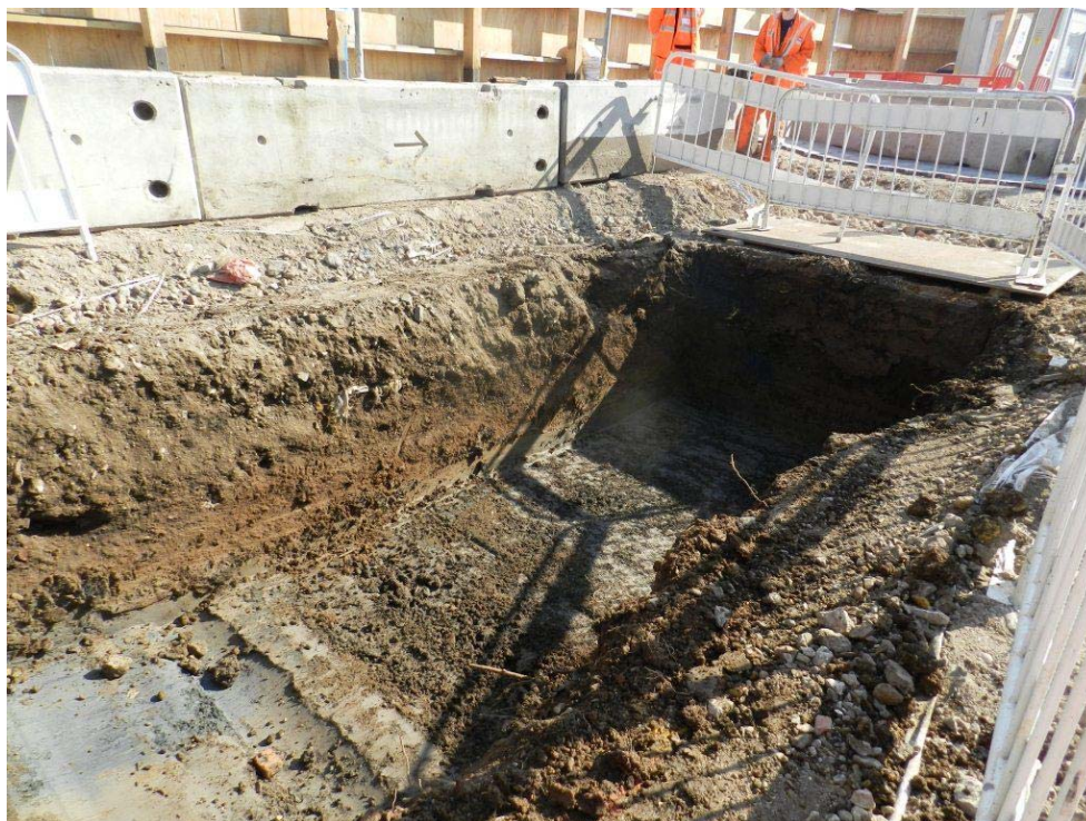
Trench 4: alluvium exposed beneath imported topsoil
