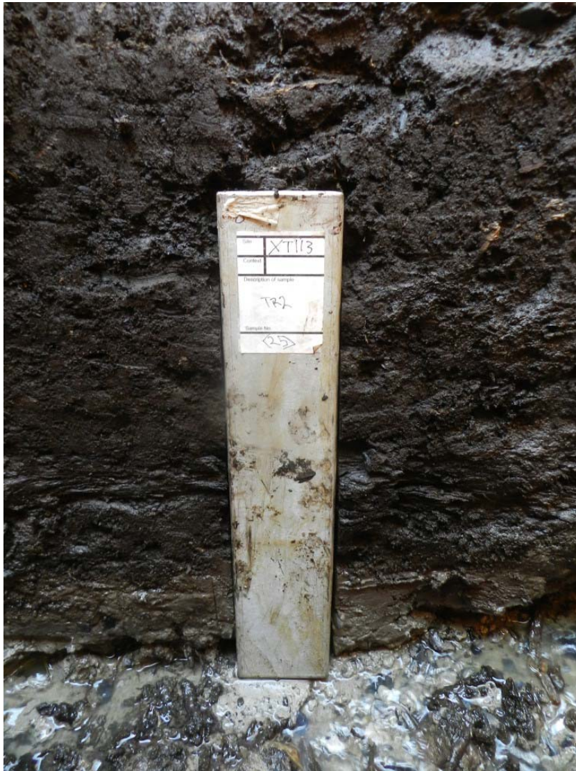
Photo 4 monolith <25> with water undermining the section
