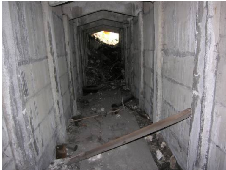
Fig 16 An internal view of shelter 2 looking east
