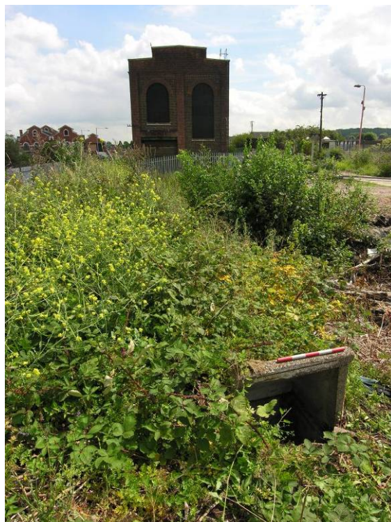
Fig 17 The escape hatch in the foreground, looking east
