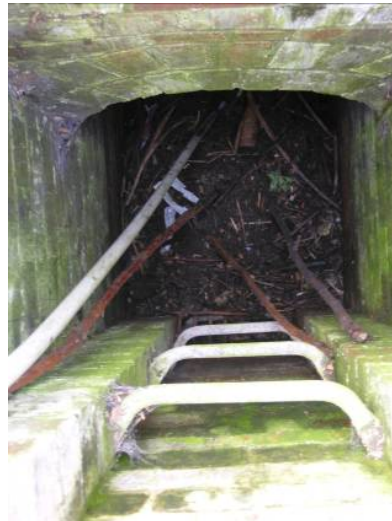
Fig 13 The escape shaft to the south of the shelter
