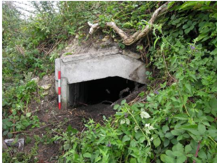
Fig 15 A view of the entrance to shelter 2 looking west
