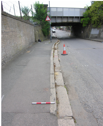
Fig 10 Kerbstones underneath NKL railway bridge on White Hart Road.
