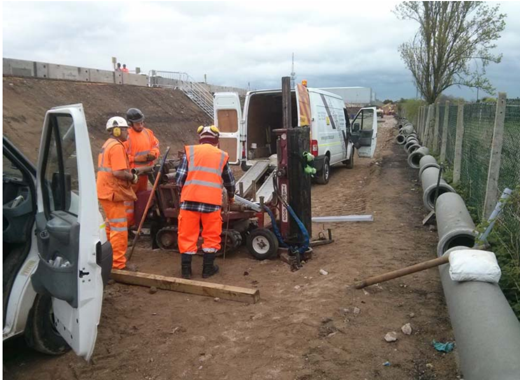
Photo 1 Borehole 7 Looking East
