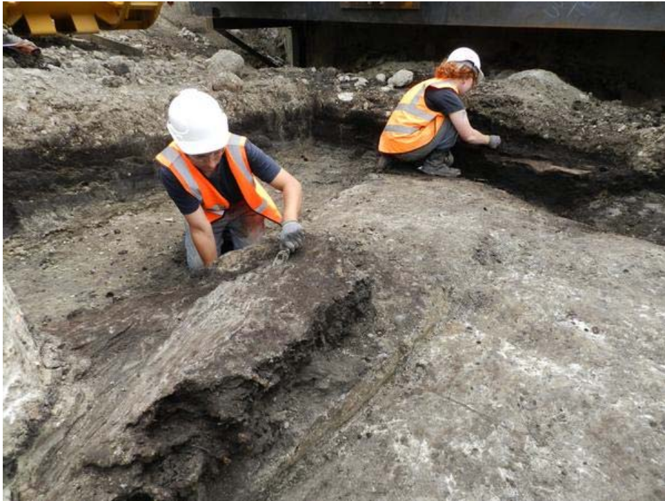
Photo 9 Trench 1D Timbers [32] (left) and [34] (right)
