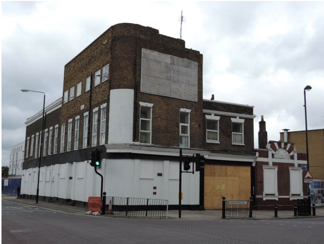
Fig 2 The Barge, looking north-west
