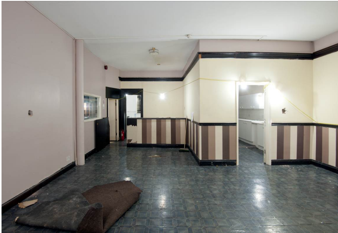
Fig 21 The saloon bar, looking west. Note the supporting column, the dado and picture rails and the moulded door architrave
