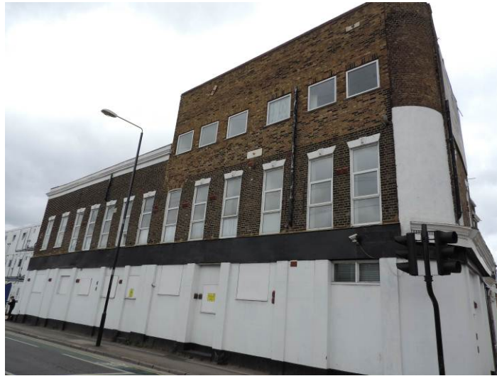
Fig 8 The southern façade of the Barge, looking north-west
