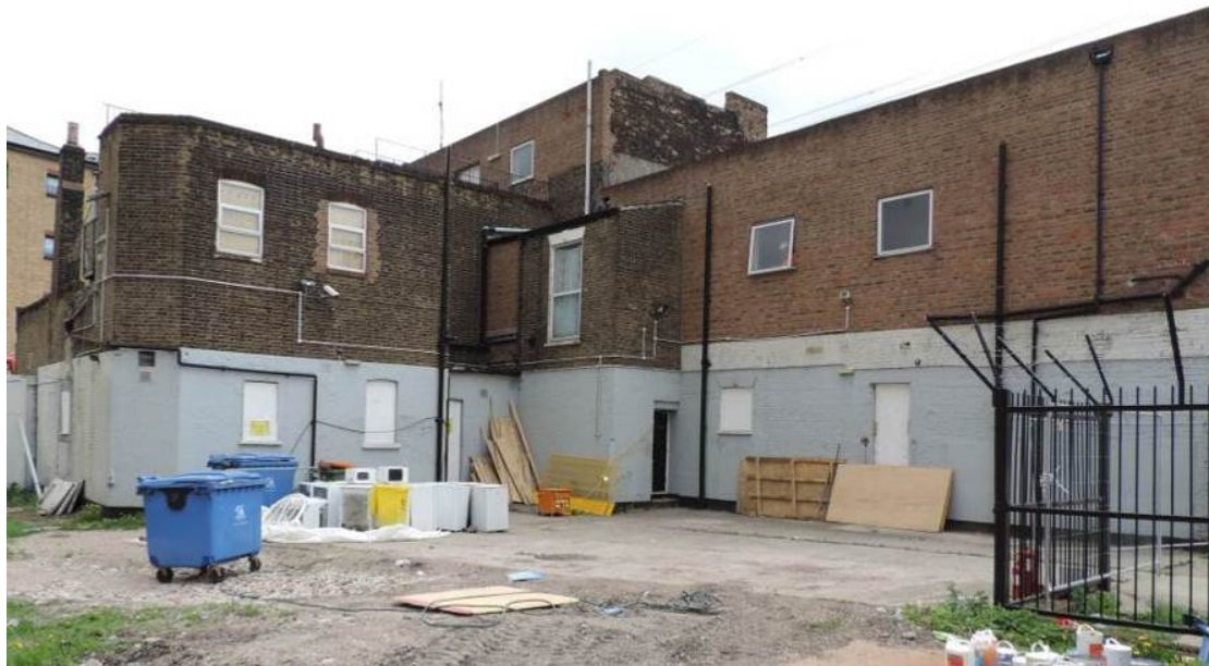
Fig 16 North and west elevation of the building, looking south-east
