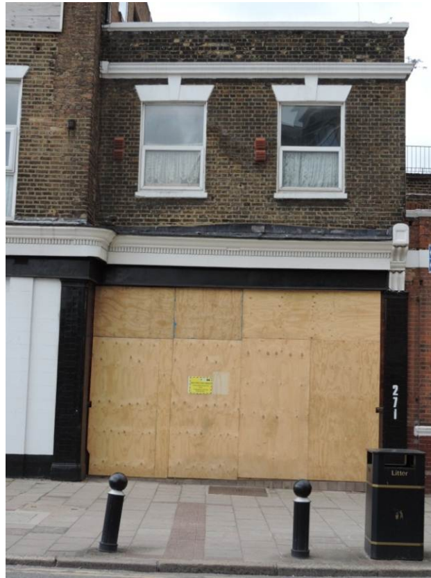
Fig 12 East elevation of the Phase 2 extension, looking west
