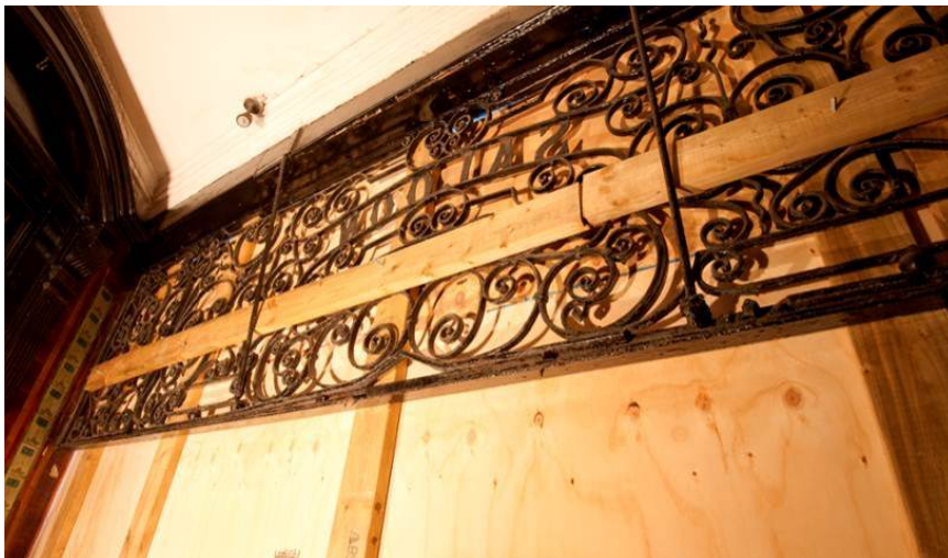
Fig 11 Open work wrought iron above the main entrance
