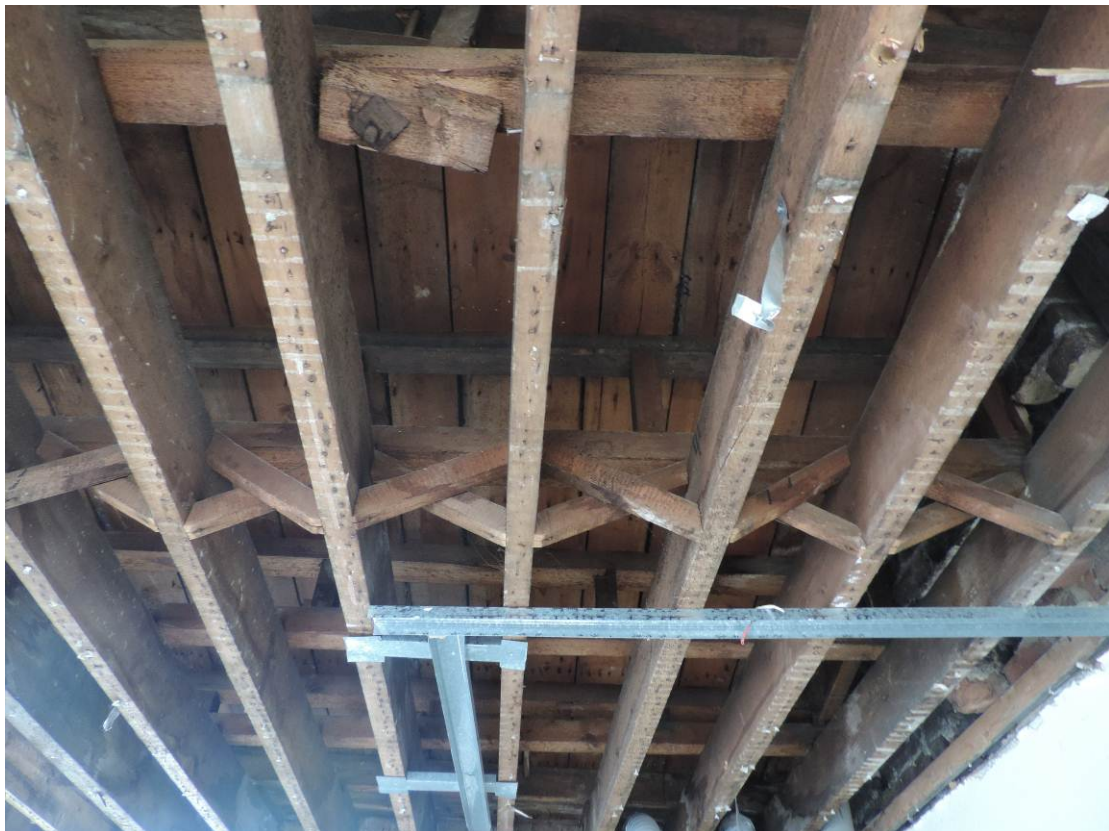
Fig 25 First floor ceiling structure, looking west
