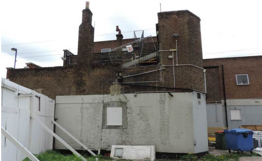
Fig 17 North facing elevation of the building, looking south
