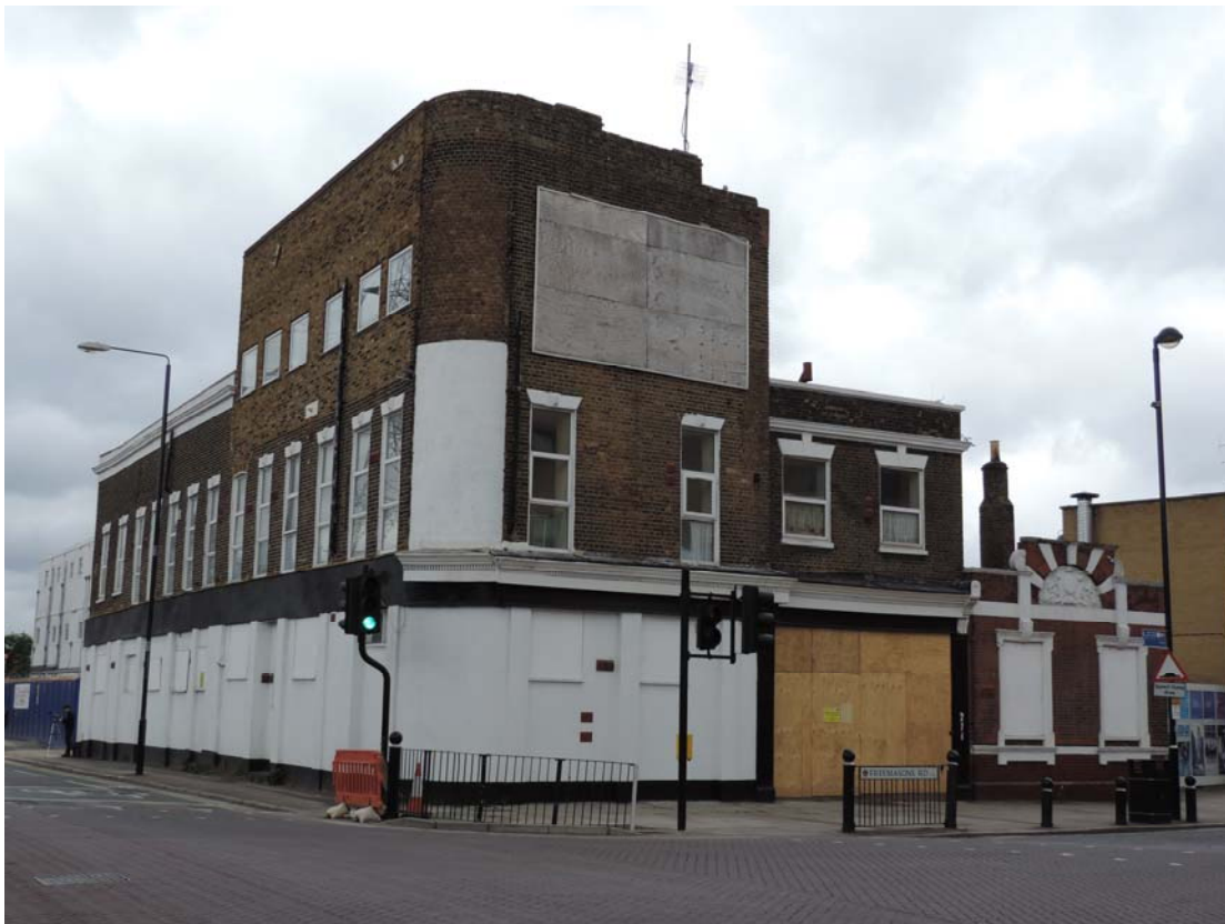
Fig 1 A general view of the late 19th century public house looking north-west
