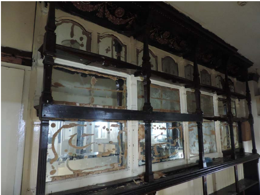
Fig 4 Spirit shelves with frosted and etched mirrors behind the timber bar, looking north-west
