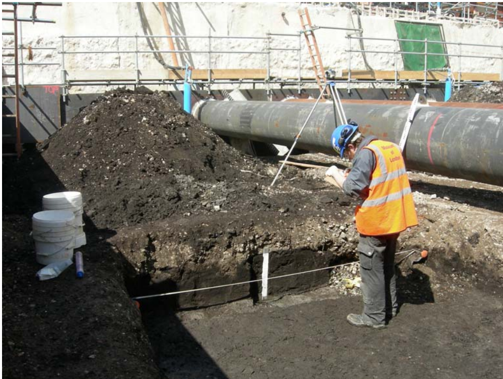
Photo 1 Sampling the peat [2] and underlying gravels [1] in Trench 1A (looking north)
