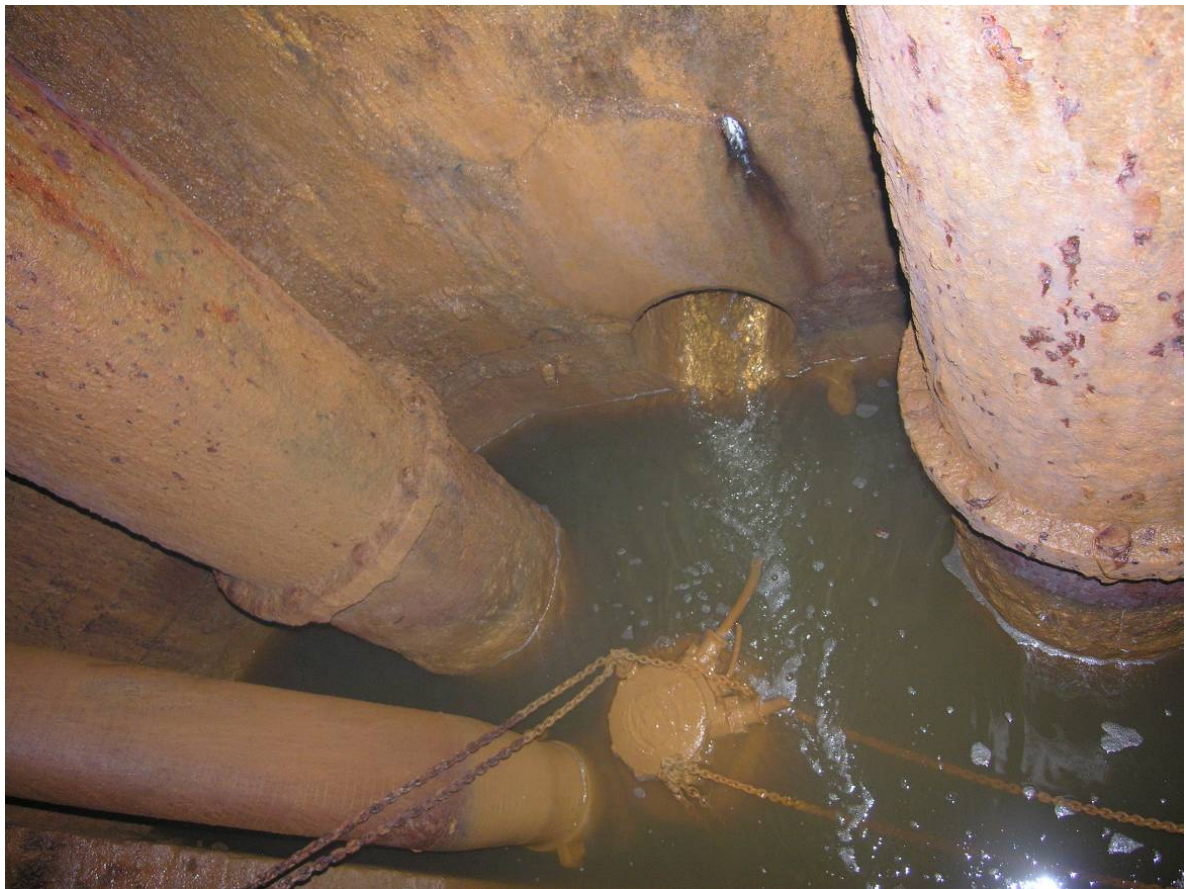
Photo 20. The base of the shaft showing the inlet with water flowing in from the Connaught Tunnel. The earlier abandoned electrical pump is partially submerged in the centre of the photograph.
