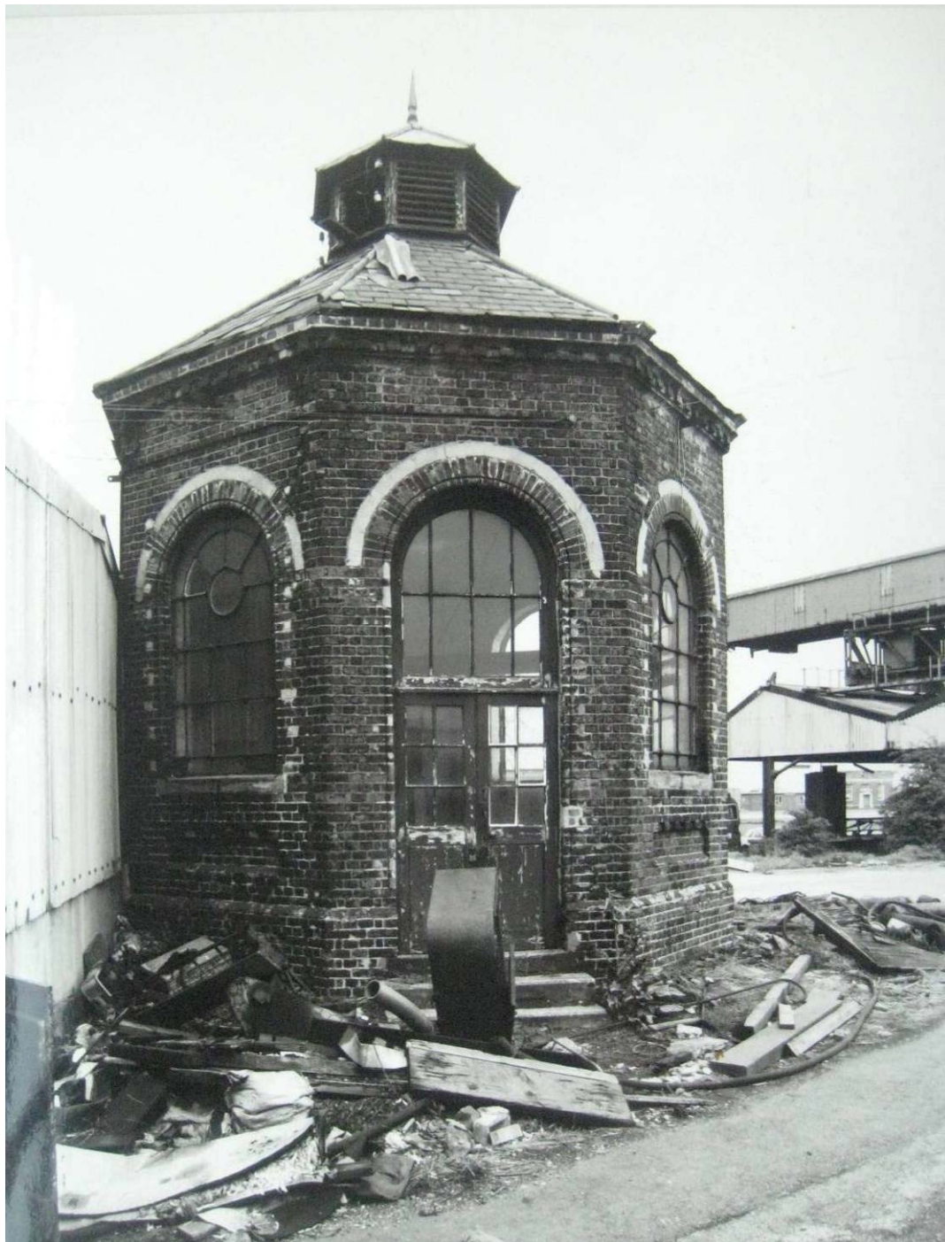
Fig 9 The pumphouse entrance from the south, taken 1977. (LMA SC/PHL/02-SSo4 0921-30)
