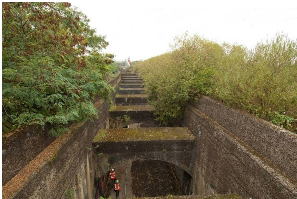
Photo 24. The buttresses of the north cutting looking west.
