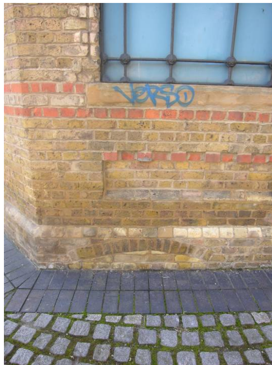
Photo 9. The single course segmental brick arch in the north western façade.
