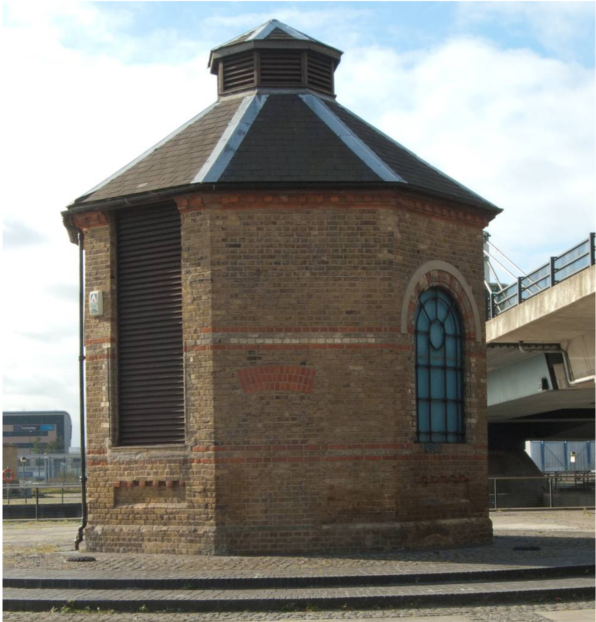
Photo 7. The north east façade with the timber louvers and the north façade with the segmental arch visible from a blocked former doorway
