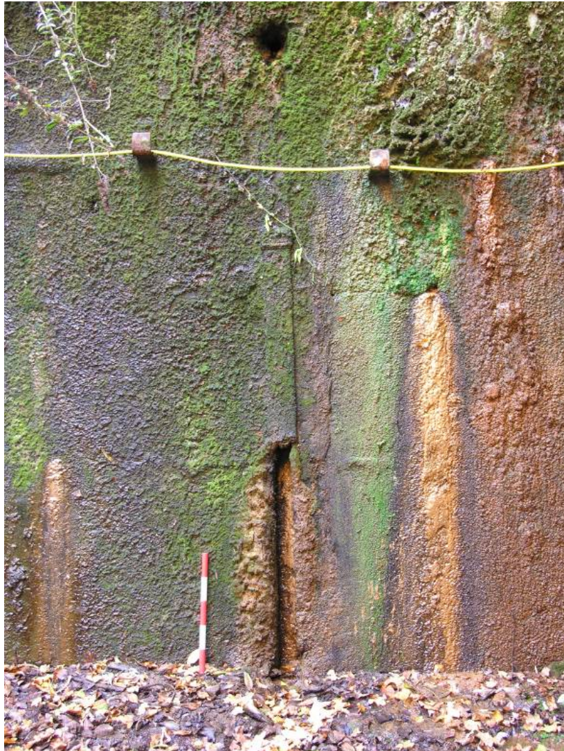
Photo 48 The recessed drain pipe outside the south portal looking south.
