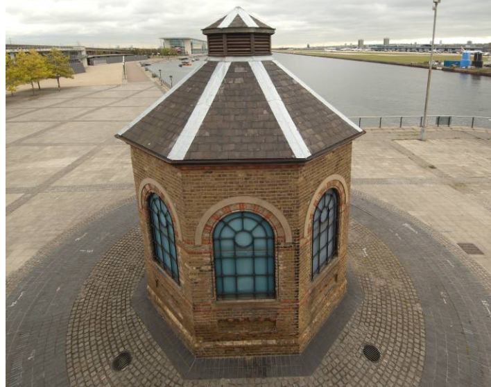
Photo 2. The pumphouse looking east from the Connaught Bridge
