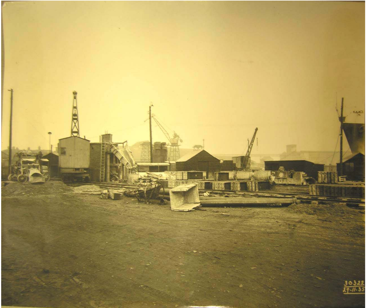
Fig 7 DSCN6814 A 1935 photograph from Museum of London Docklands showing access to the tunnel works via the via southern ventilation shaft in the left of the photo next to the crane. (MLDSSC 23896 – Album B)
