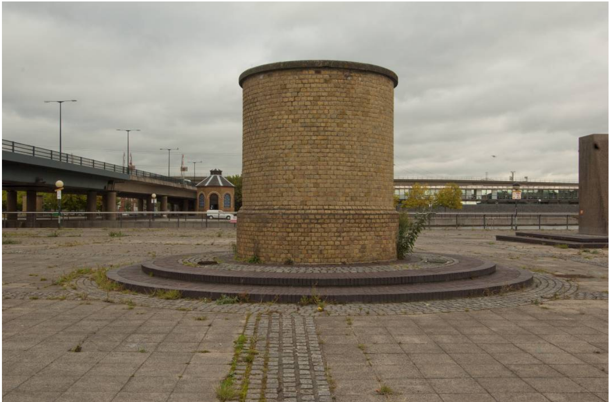
Photo 21. The southern air vent structure with the pumphouse in the background, the northern air vent is just visible behind the Connaught Bridge in the far left of the photo.
