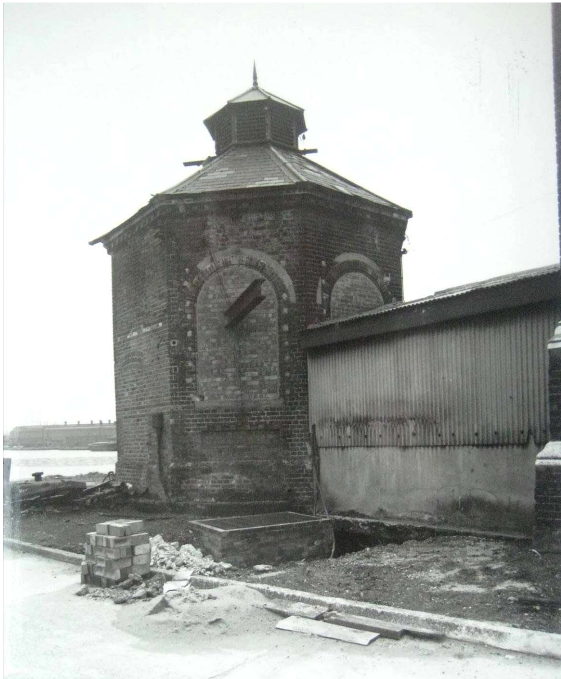
Fig 11. The north-western elevation looking south east, taken 1977. (LMA SC/PHL/02-SSo4 0921-31)
