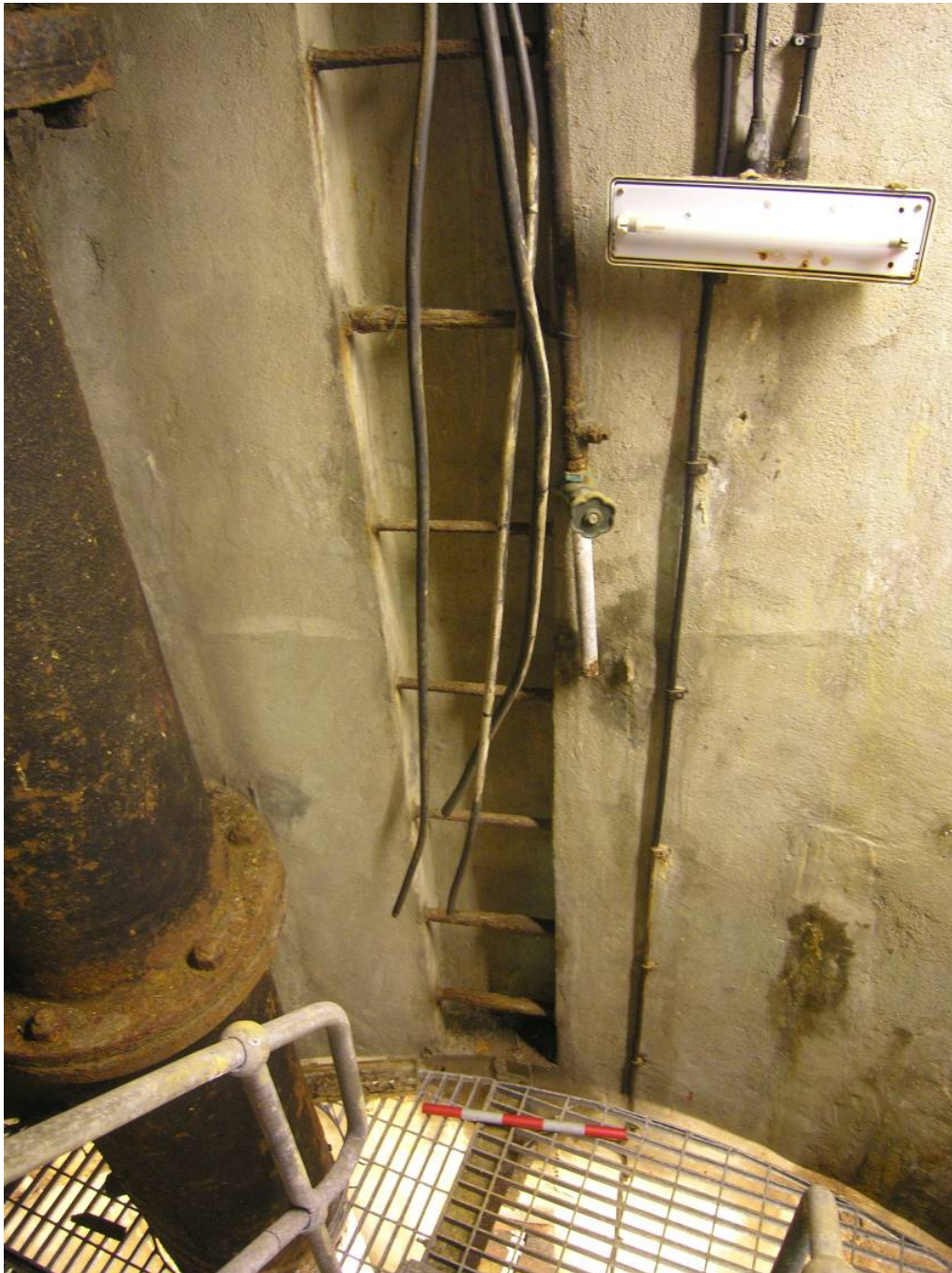
Photo 17. The original step ladder access into the shaft, set within a recess in the western side of the shaft wall, looking west.
