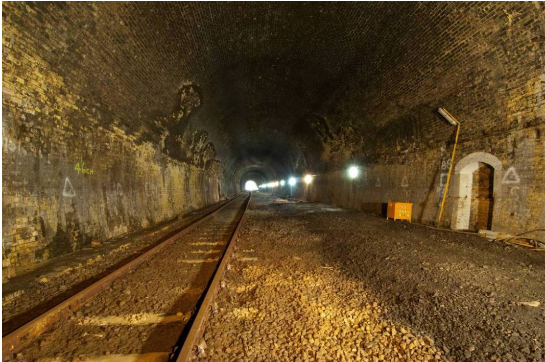
Photo 40 The view south down the southern brick single section of tunnel.
