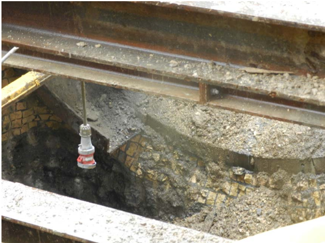
Photo 56 Masonry below the steel rings
