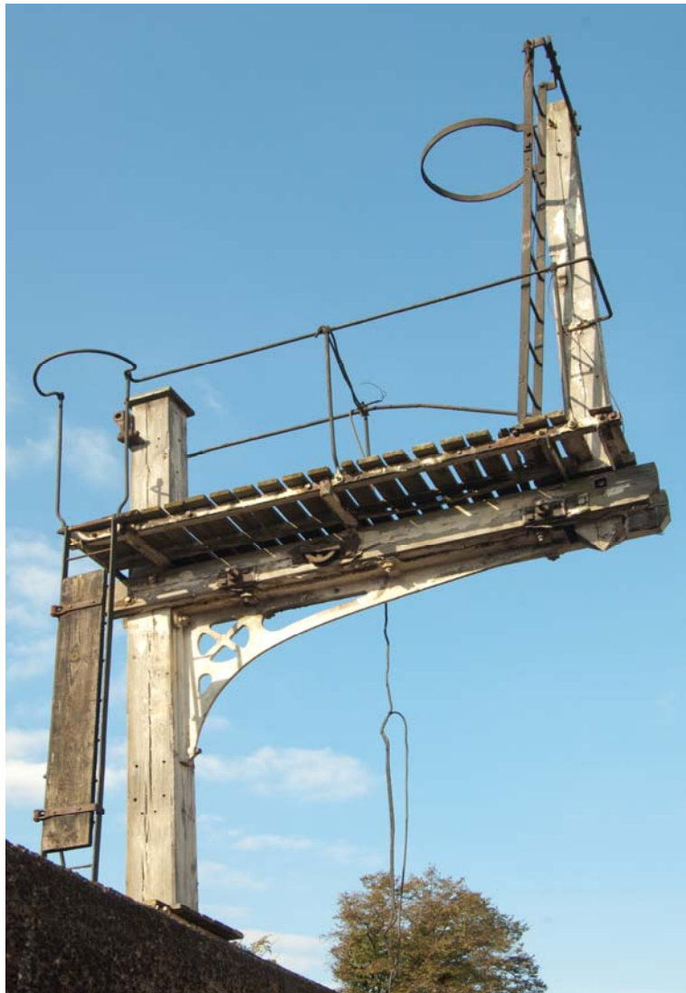
Photo 45 The gallows signal at the southern end of the south cutting looking north west.
