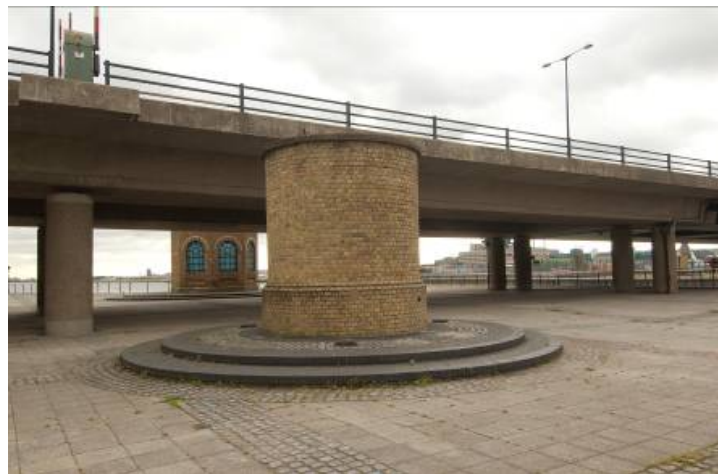
Photo 3. The air vent on the north side of the Connaught Passage looking east, with the pumphouse in the background.
