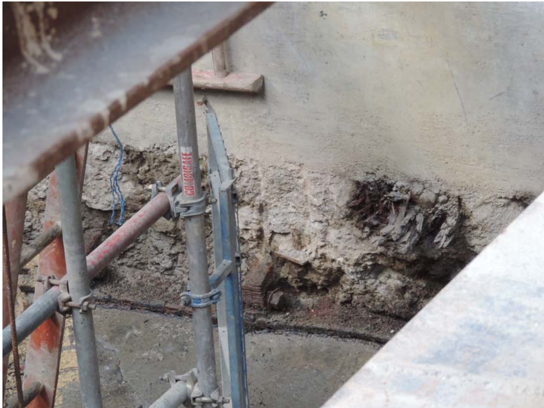
Photo 55 Timbers encased in concrete possibly relating to the former trackbed
