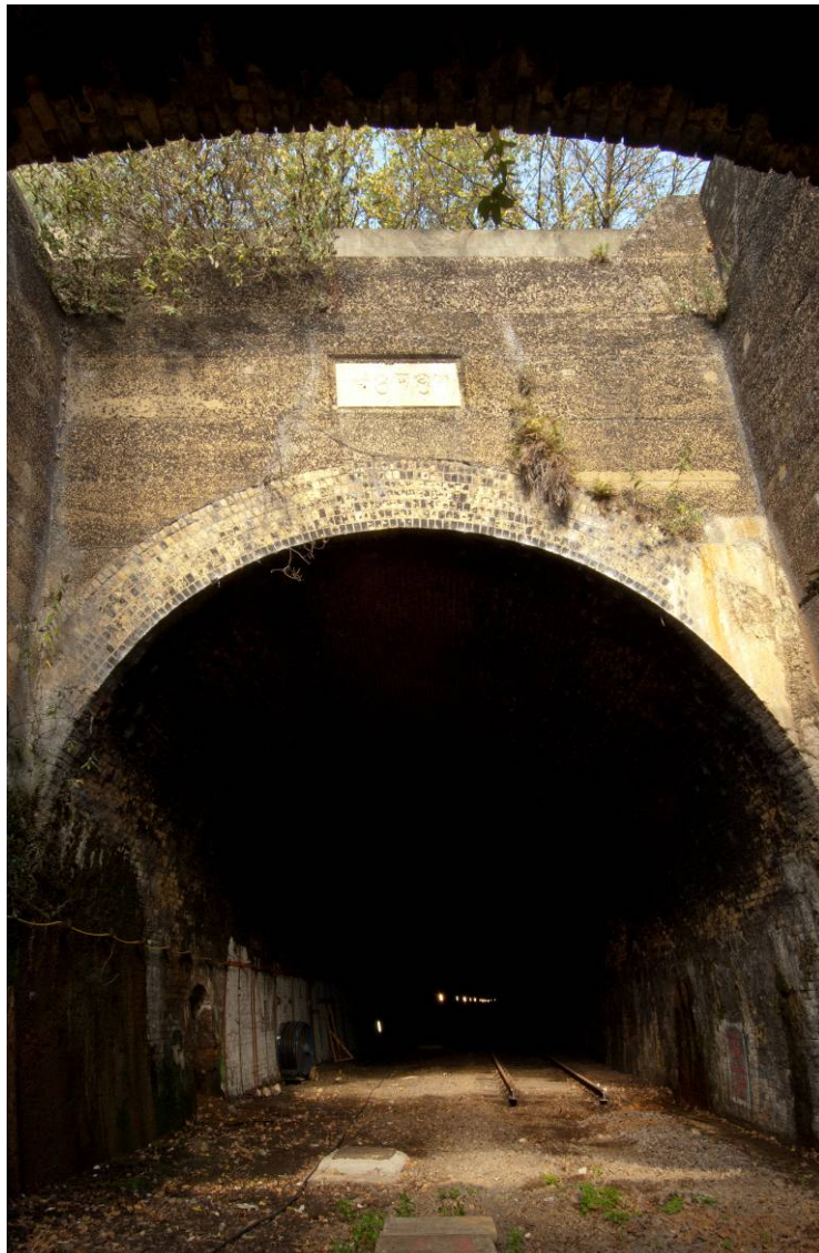
Photo 42 The south portal looking north.
