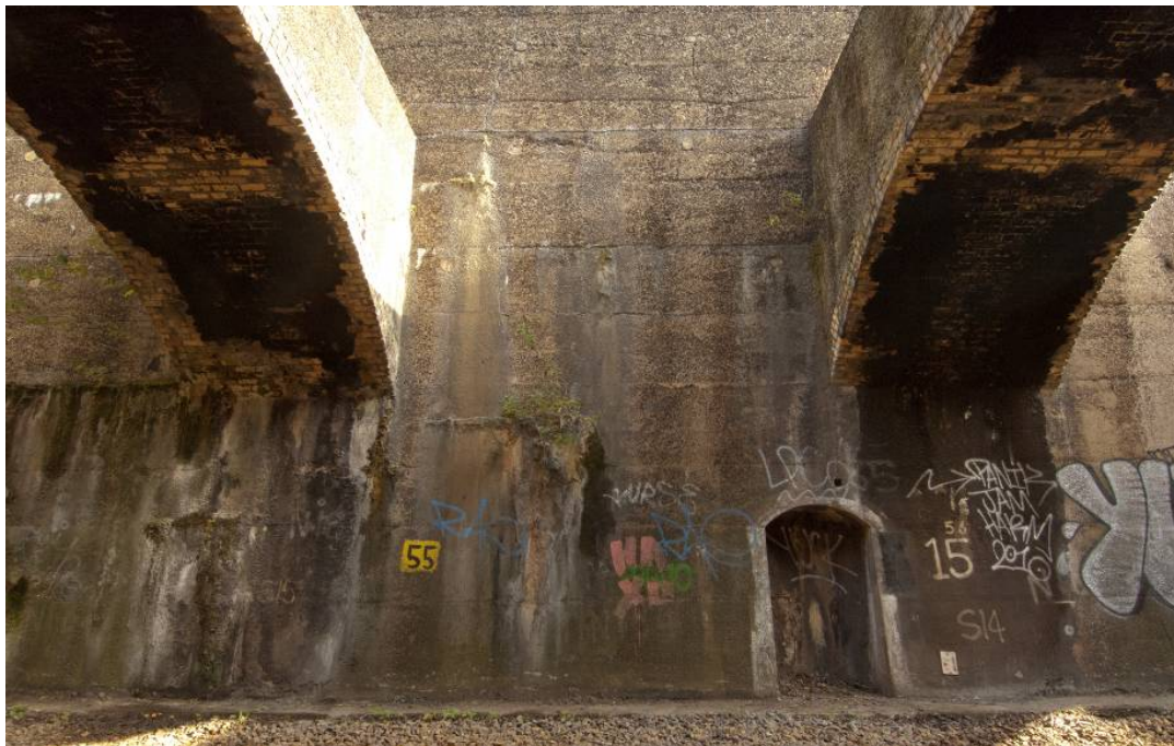
Photo 44 Arched buttresses in the southern cutting, looking east.
