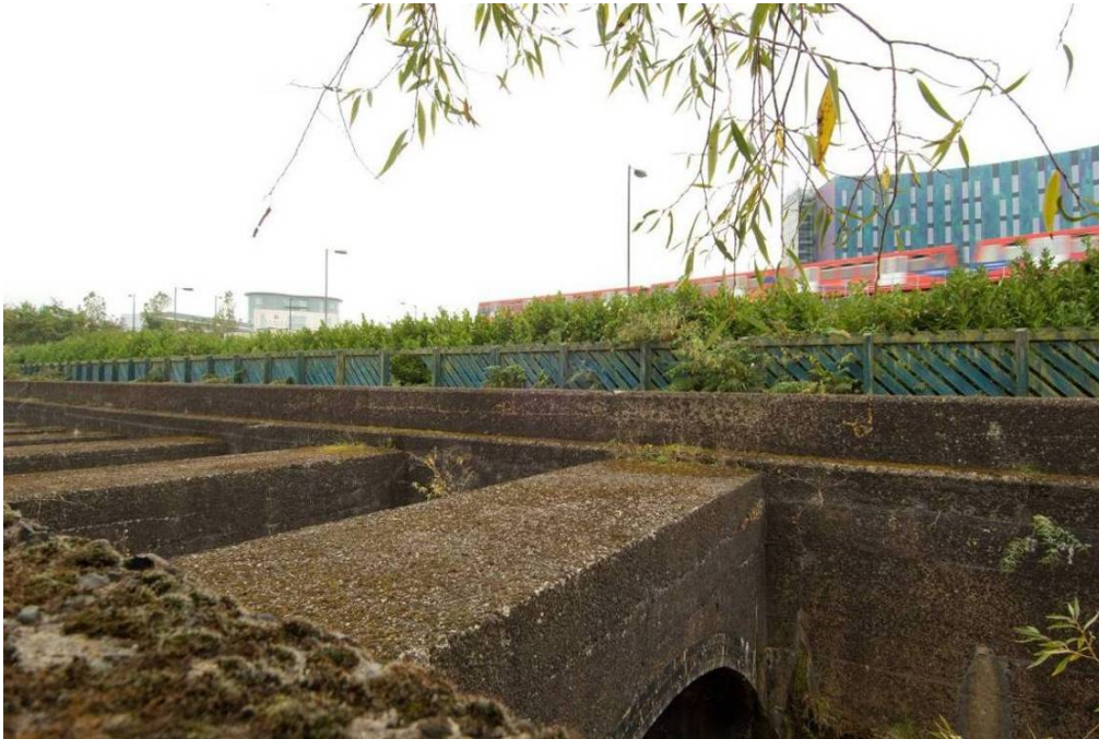
Photo 23. The first or westernmost of the arched buttresses in the approach to the north portal looking south east. Note the gradual increase in depth of the buttresses to the left.
