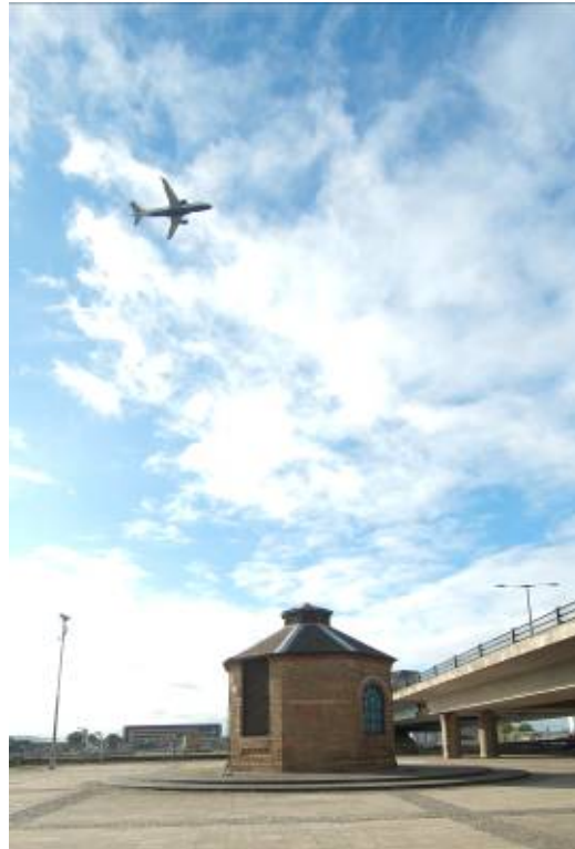
Photo 4 The pumphouse looking south.
