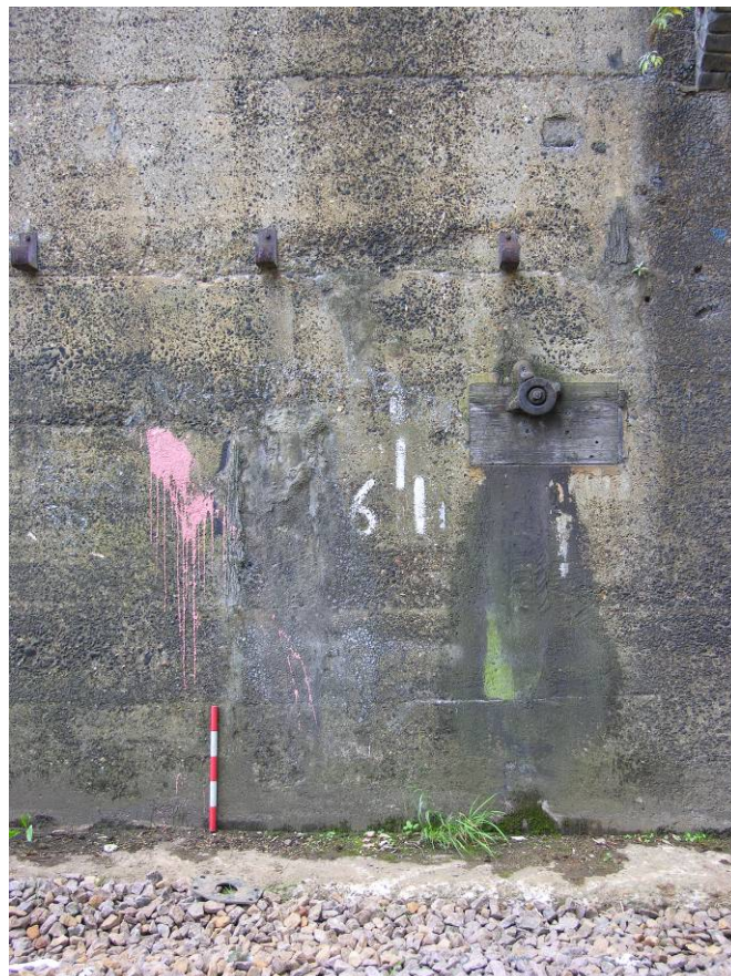
Photo 47 The larger pulley wheel mounted on timber, set into the cutting wall, looking south.
