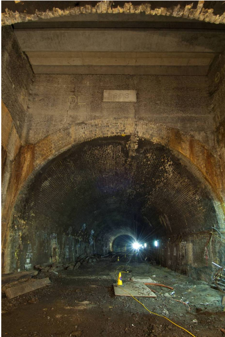
Photo 27 The north portal of the tunnel, looking east.
