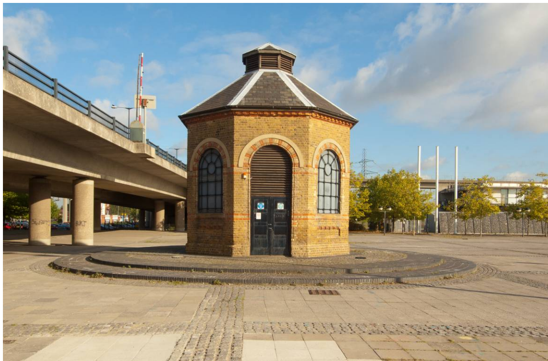
Photo 5. The entrance and southern façade of the pumphouse looking north
