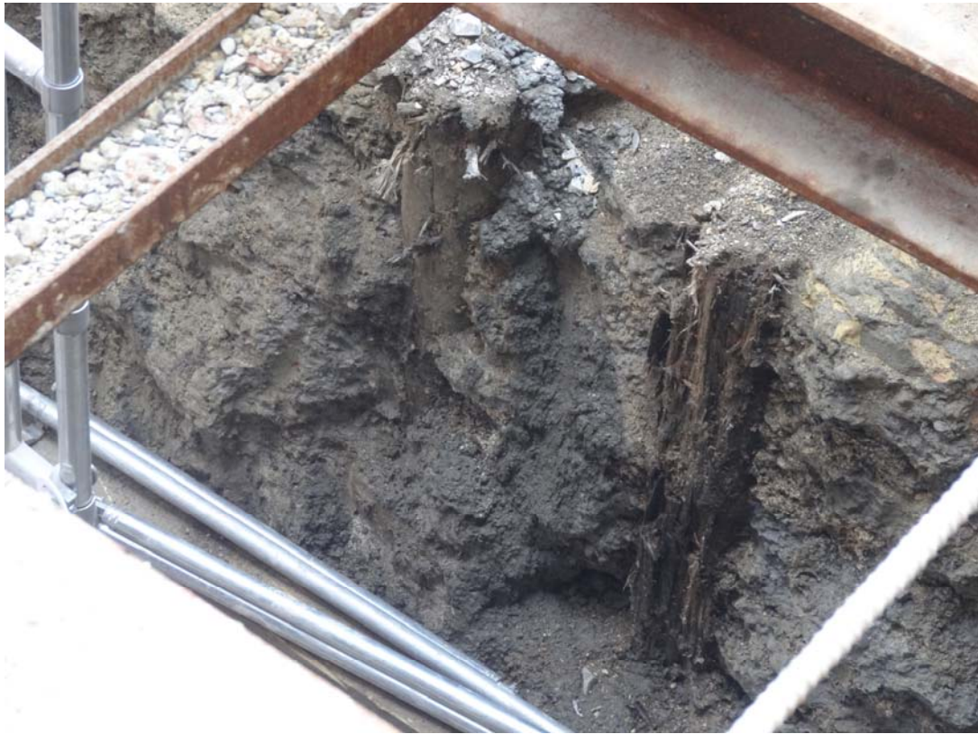
Photo 57 Timber posts supporting masonry of the 1870s construction
