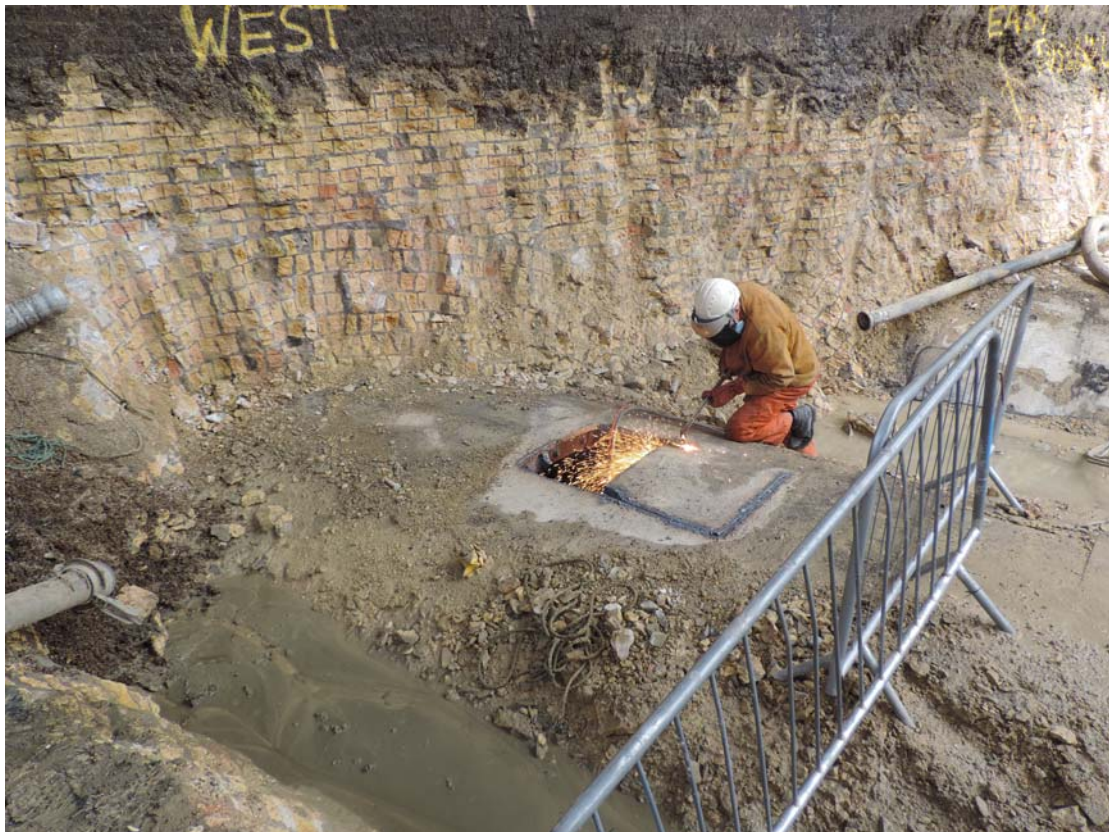
Photo 53 Removal of the upper section of the steel rings
