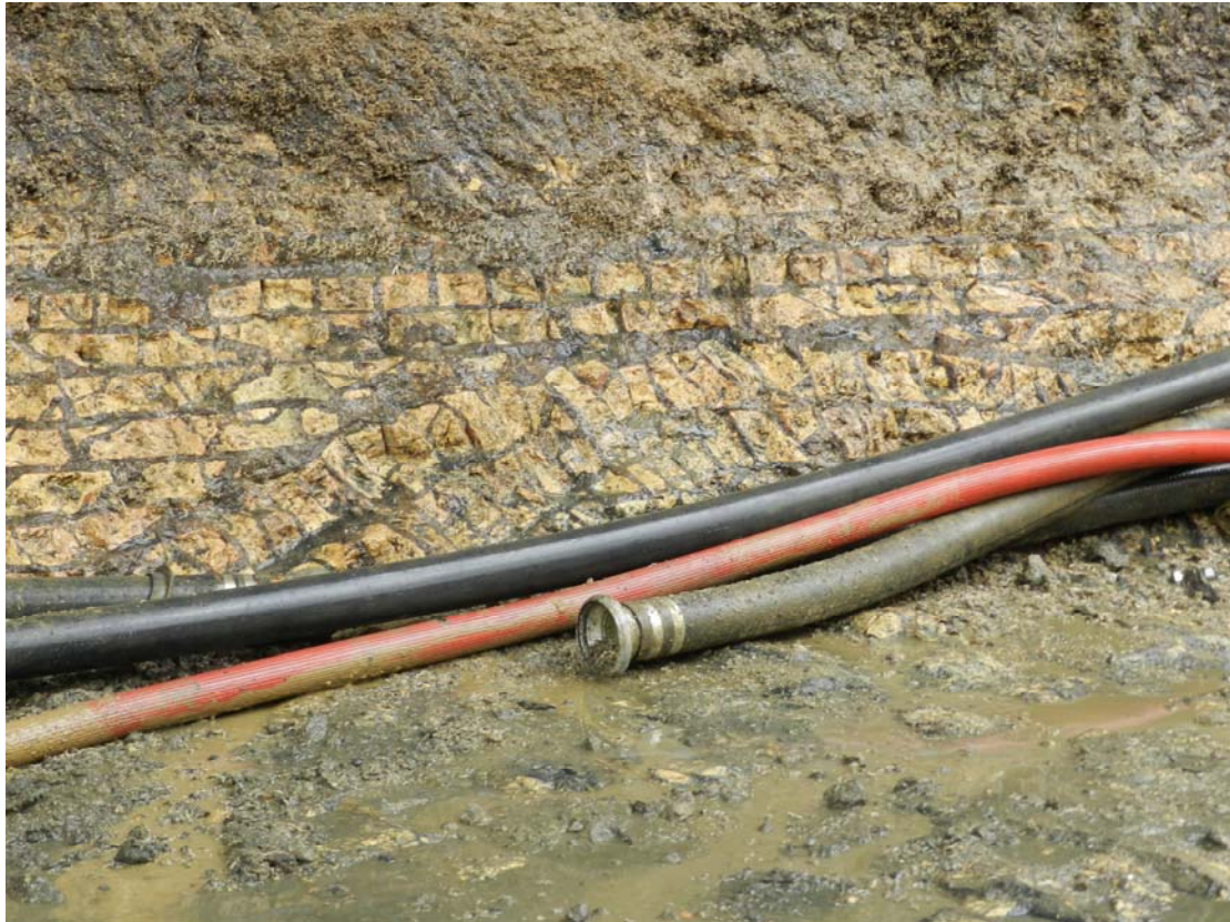
Photo 52 Brickwork at the bottom of the Connaught Passage
