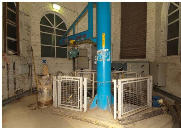
Photo 15. The interior of the pumphouse looking north showing the modern hoist.
