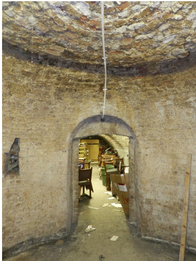
Fig 12 Doorway of the Beehive, view from inside, looking north.
