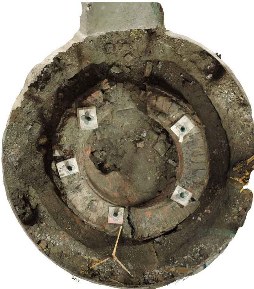
Fig 27 Plan view of the revealed brick structure in the Beehive.
