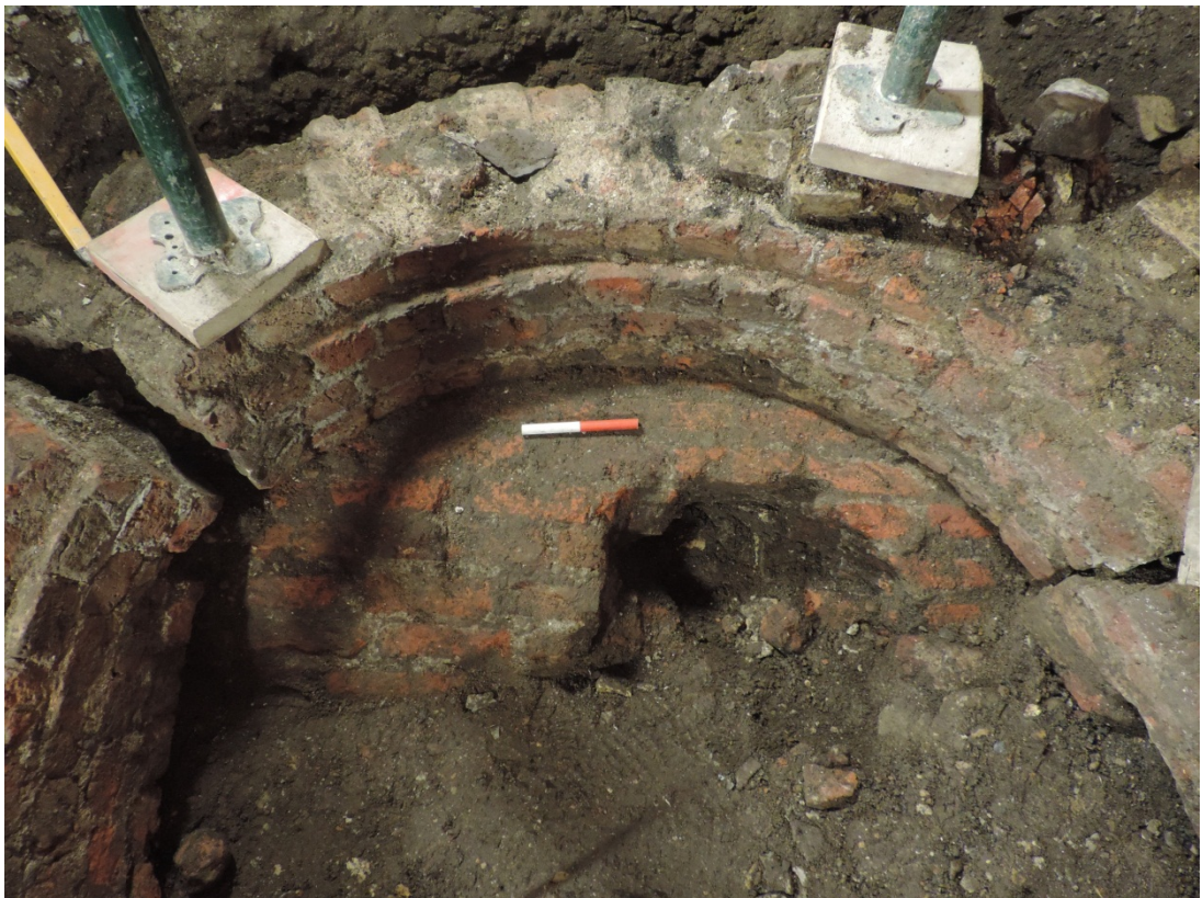
Fig 15 Circular brick wall constructed on 1772 brick built sewer, looking west
