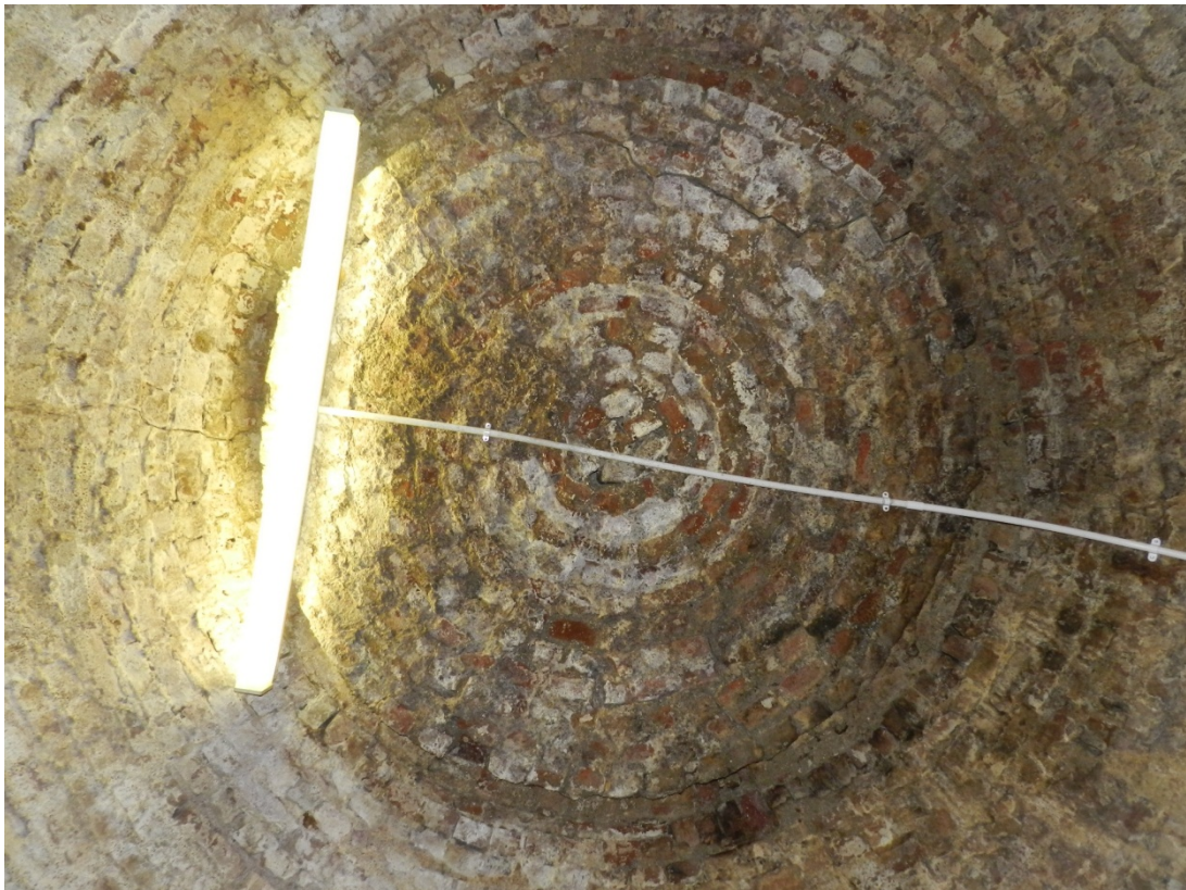
Fig 10 Circular plug or cap of the Beehive dome, looking up.
