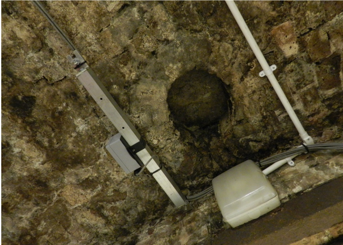
Fig 21 Circular opening in the vault (Coal chute?), looking up.
