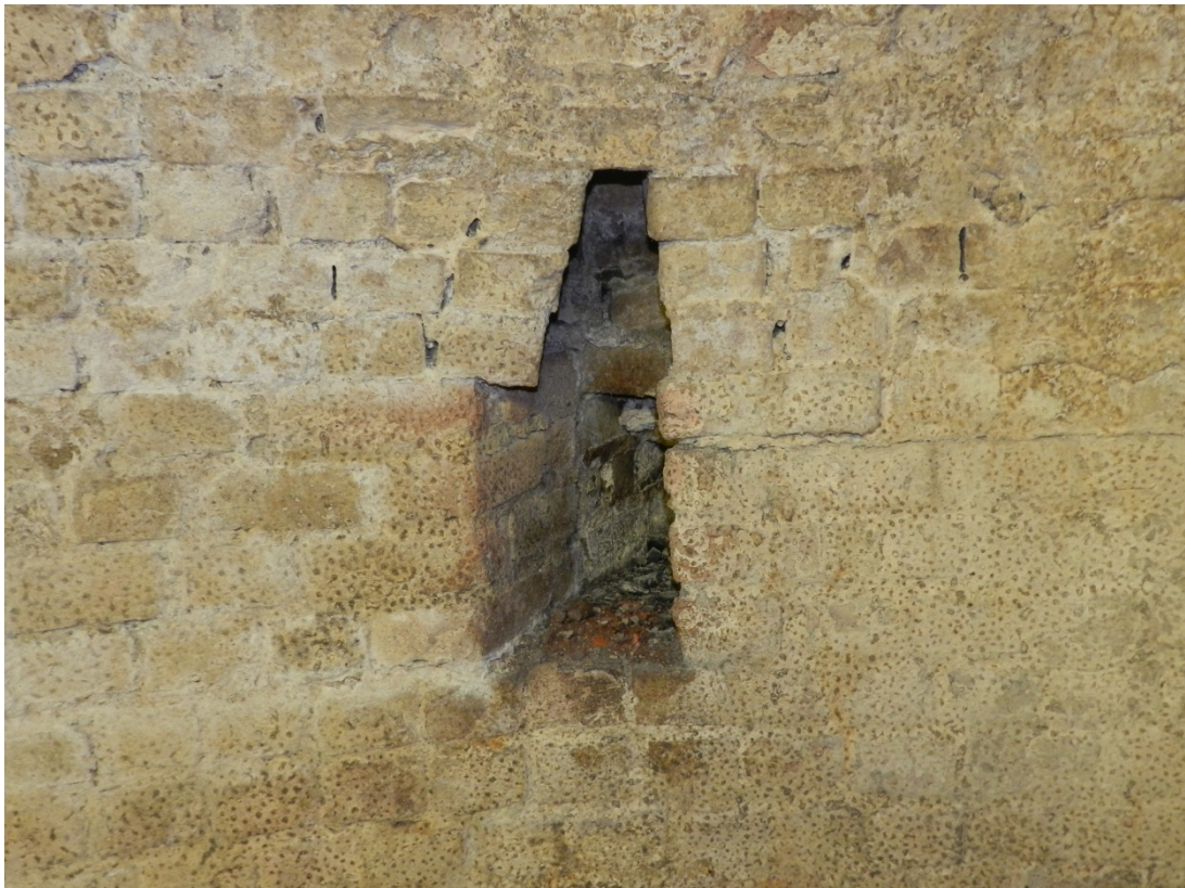
Fig 13 Small opening in the wall of the Beehive, looking north-west
