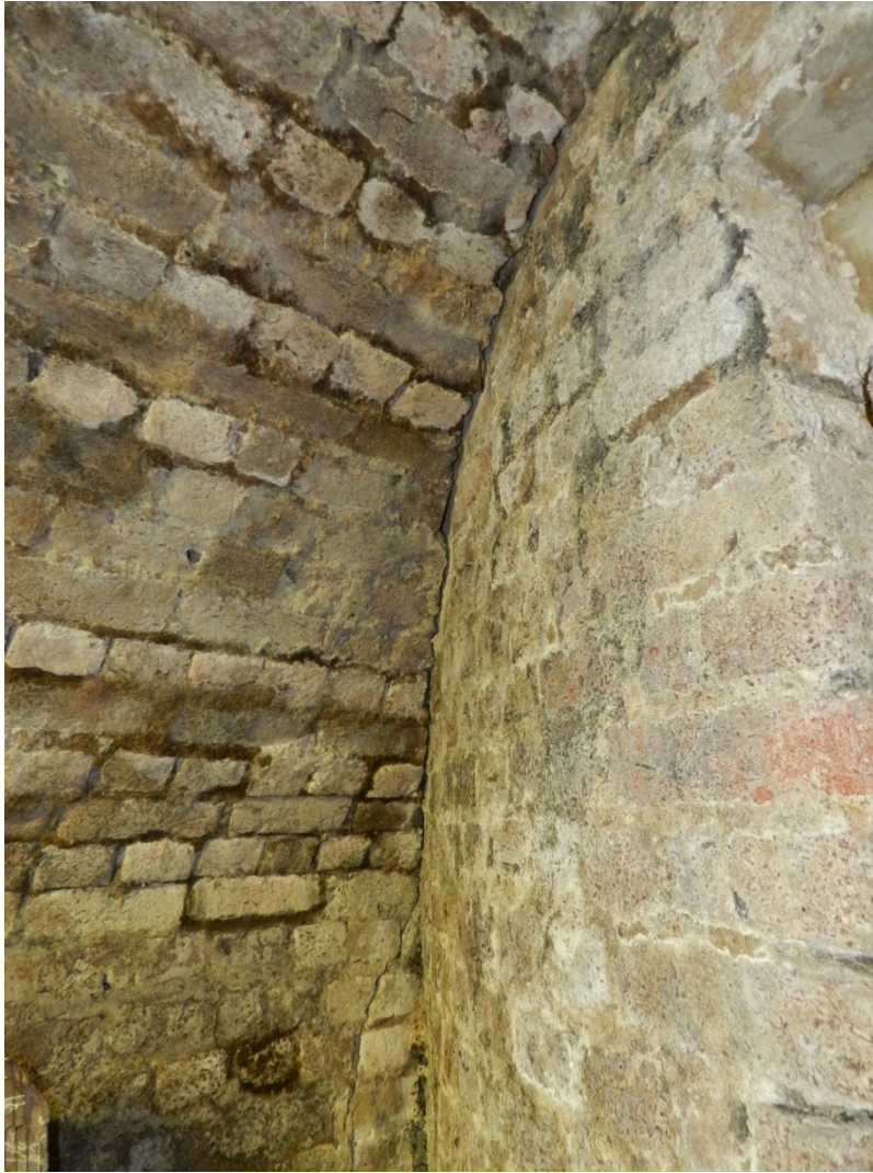
Fig 22 The eastern wall of the Barrel Vault abuts the Beehive exterior (looking south-east)
