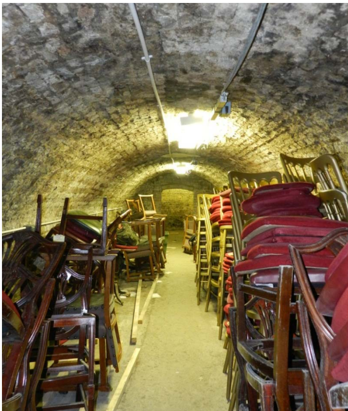
Fig 18 Interior of the Barrel Vault (looking south)
