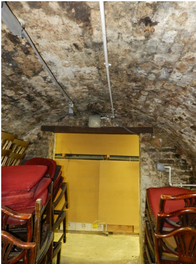
Fig 19 Access door to the Barrel Vault, internal view (looking north)
