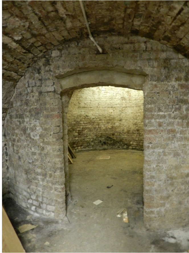
Fig 11 Access doorway to the Beehive, looking south
