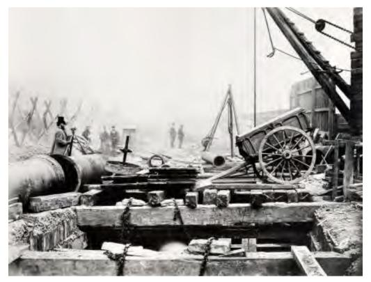
Figure 2. Photograph of the cut and cover construction of the Metropolitan Line extension to Kensington c. 1867 (Collection of the London Transport Museum)
