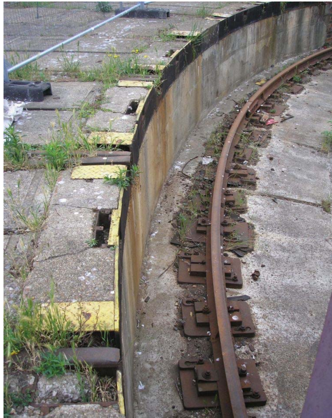
Plate 7. Metal edged turntable pit with locking pin fittings and track.
