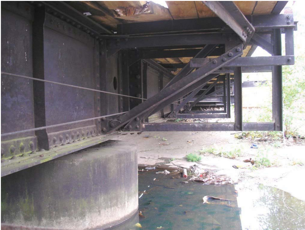
Plate 11. Underside of turntable showing supports for timber platform.
