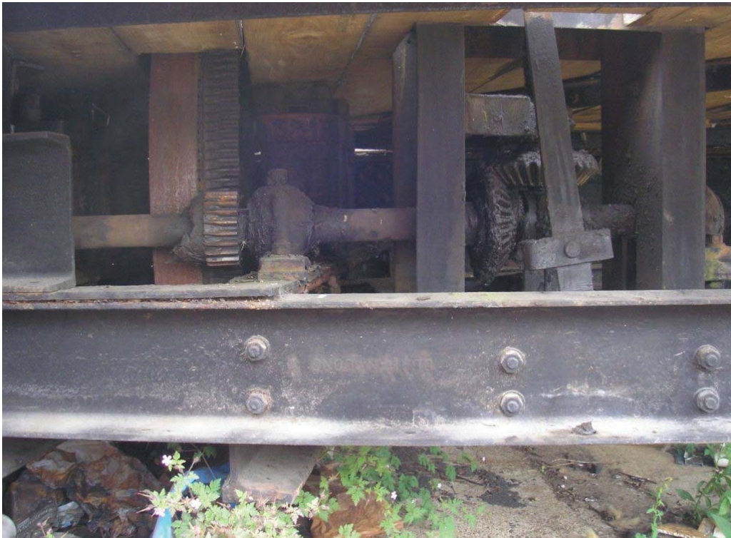
Plate 19. Turntable drive wheel linked to the hand crank mechanism. The horizontal girder in the foreground is marked with the maker's stamp 'Dorman Long Middlesbrough'.
