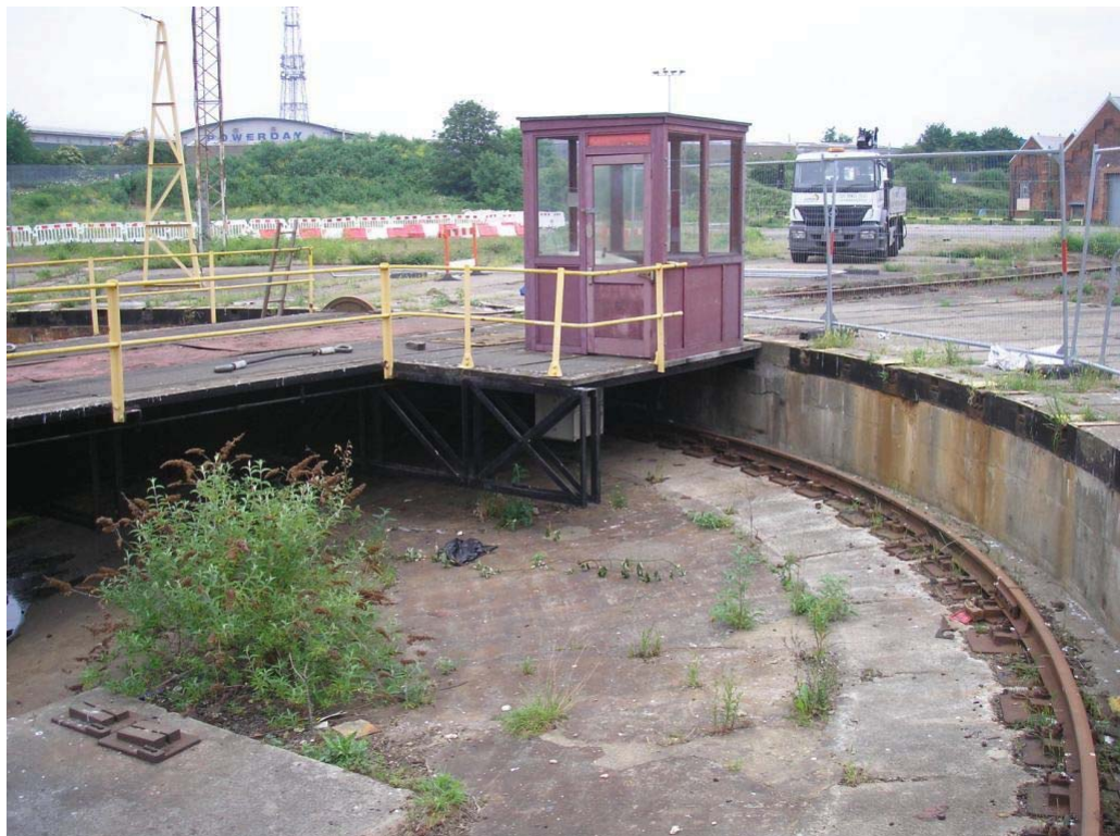
Plate 22. Operator's electric drive motor operator's booth on turntable platform.
