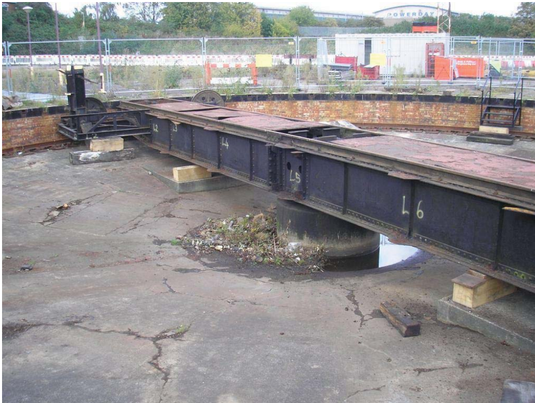
Plate 32. Turntable (left side) with deck and deck framework removed.
