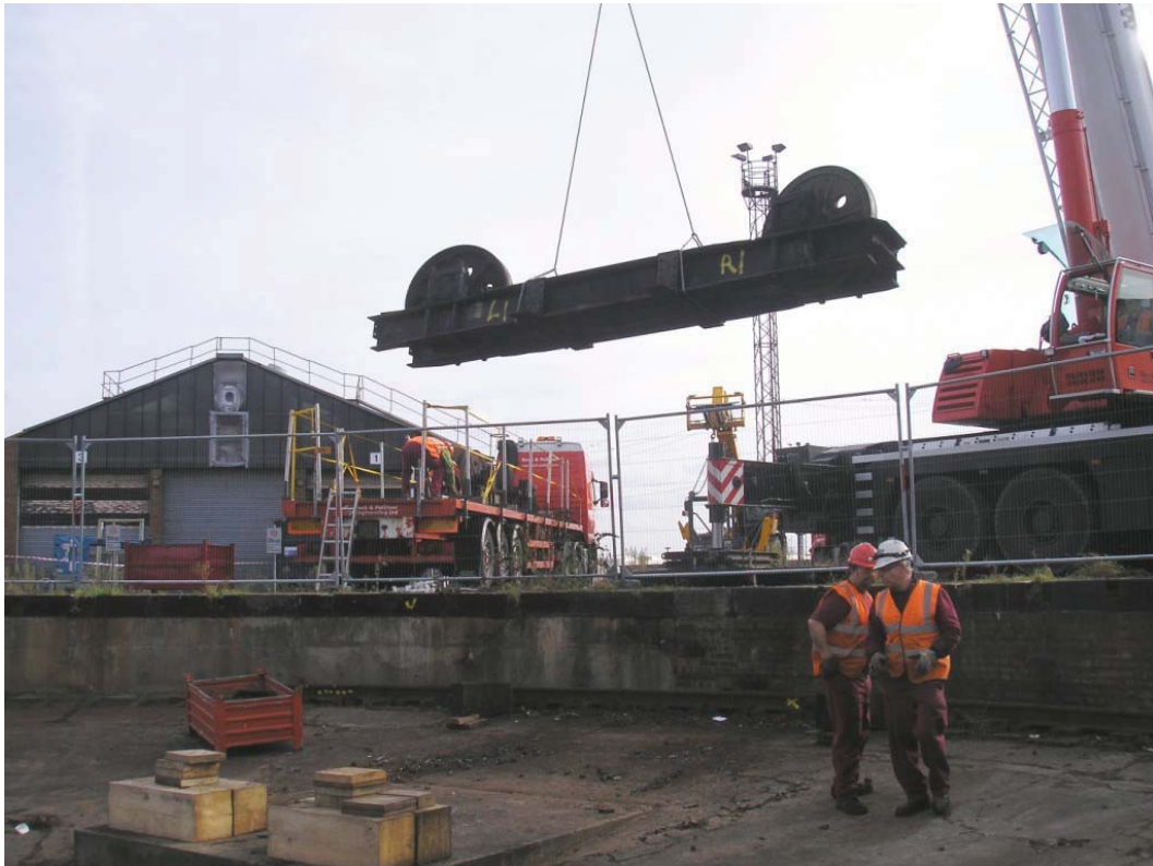
Plate 59. 'Manual' drive bogie being lifted onto a waiting lorry.
