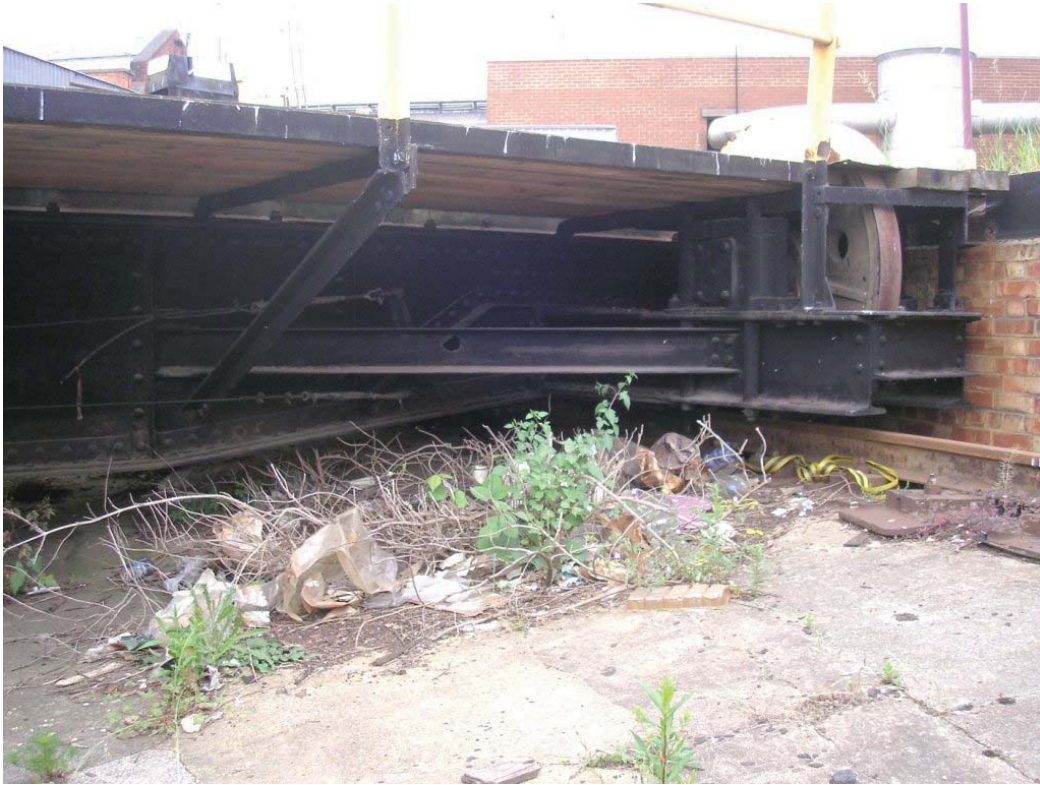
Plate 15. Turntable wheel, supporting structural elements and cables of locking bolt mechanism.
