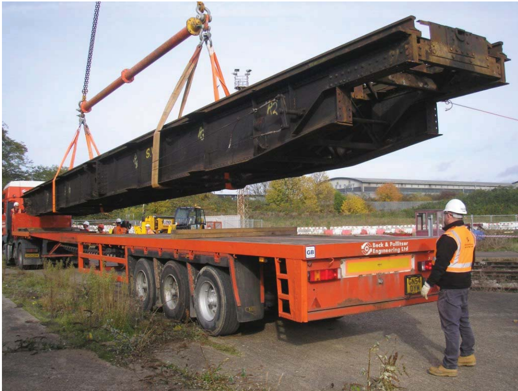
Plate 53. Turntable being lowered onto lorry.
