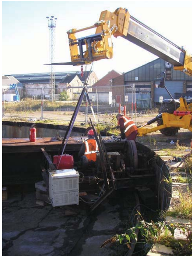
Plate 41. Electric drive unit being prepared for lifting.
