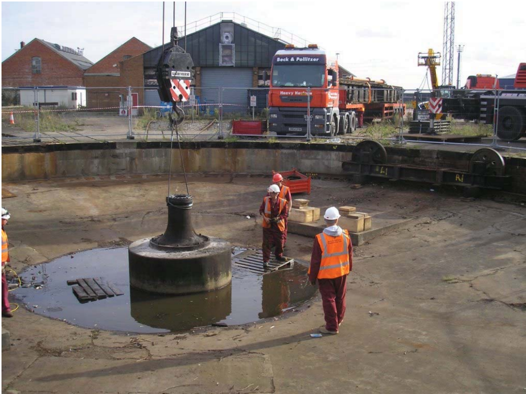
Plate 57. Pivot being lifted from concrete base.
