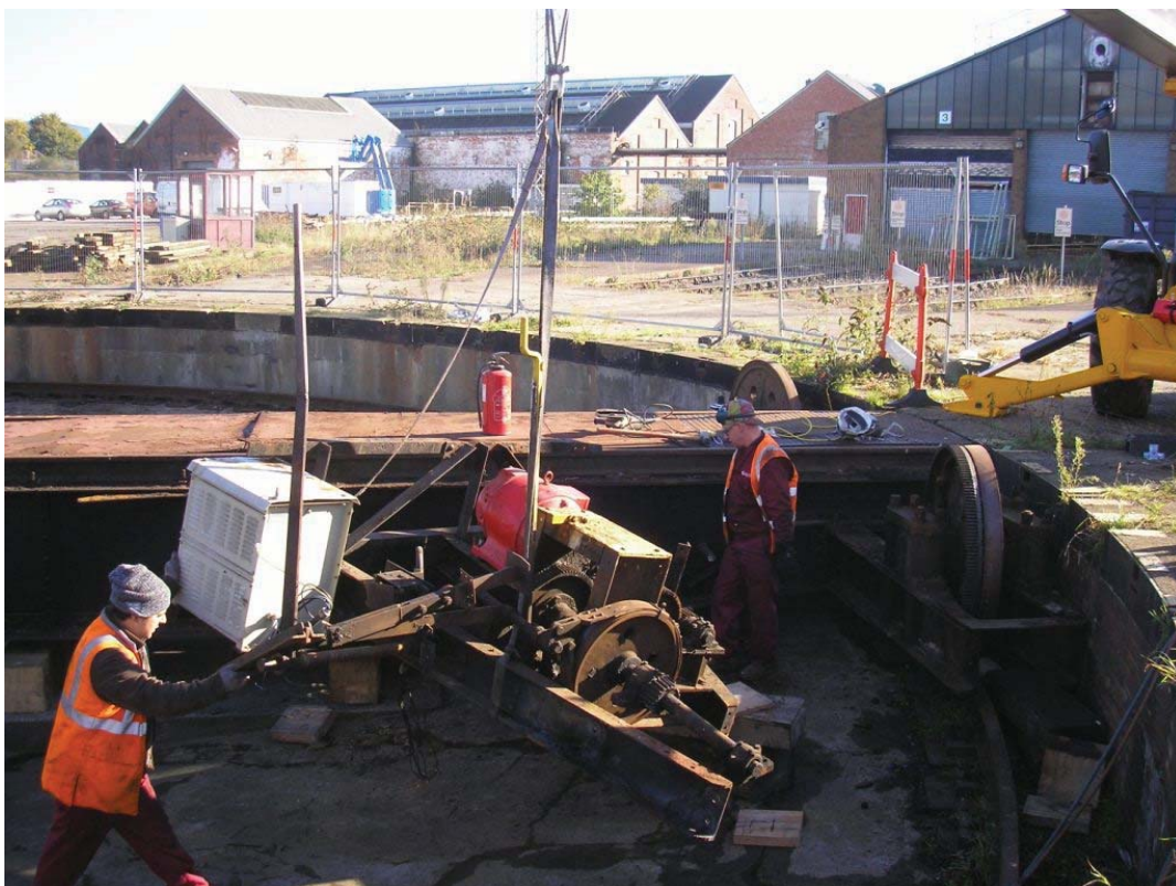
Plate 42. Electric drive unit being lifted clear of turntable in one piece.
