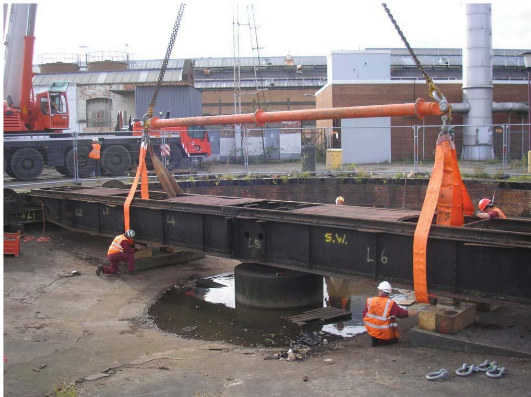
Plate 50. Turntable with straps being fitted in preparation for lifting.
