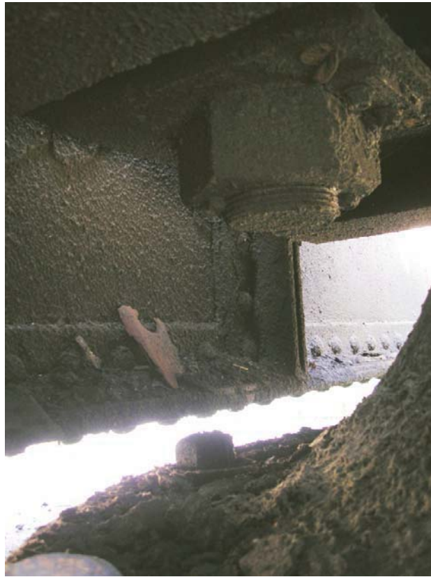
Plate 31. Base of central pivot and large bolt of turntable structure.
