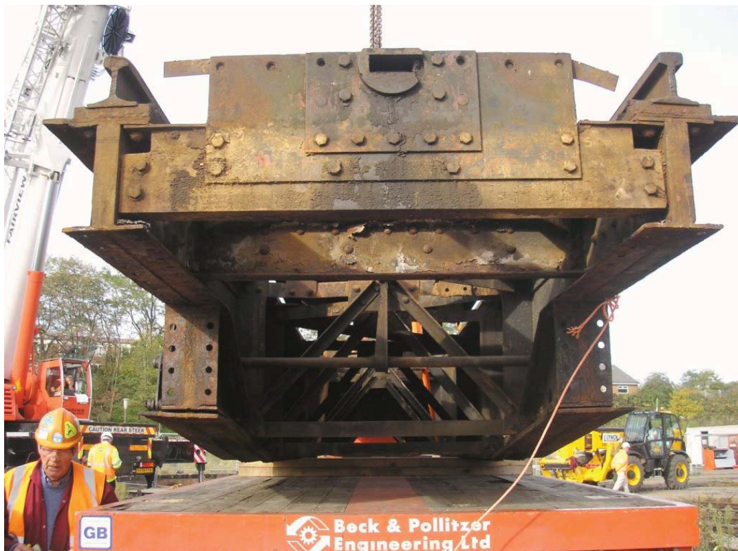
Plate 54. Previously unseen end of turntable showing rectangular slot for locking bolt at top, diagonal internal bracing, horizontal locking bolt shaft and connecting vertical arm and bolt holes for bogies.
