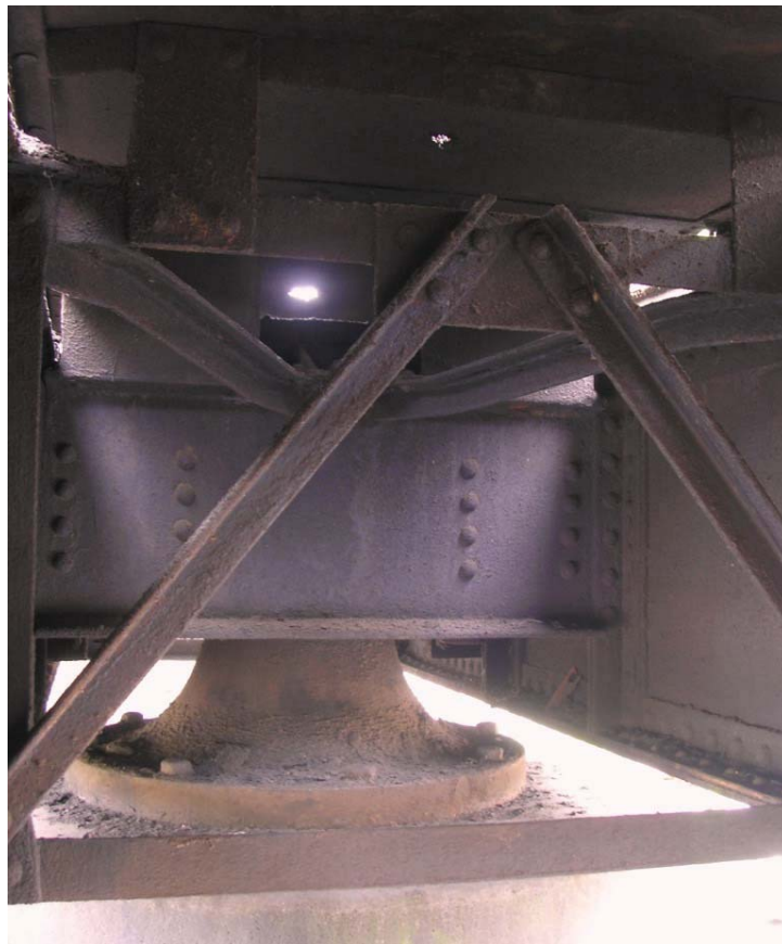
Plate 12. Underside of turntable between main beams showing central pivot.
