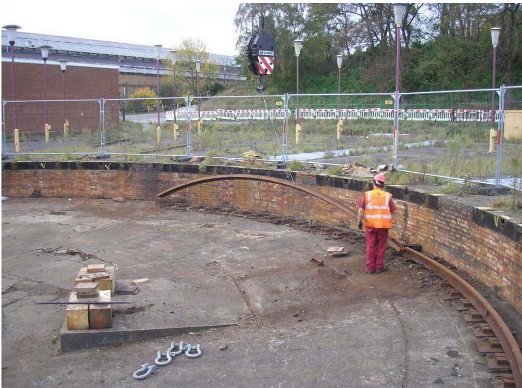
Plate 62. Turntable pit rail being lifted.
