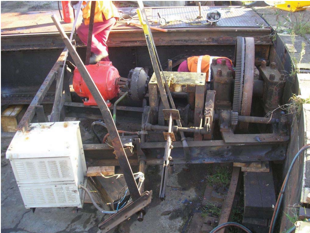
Plate 39. Electric drive unit exposed after deck removed.
