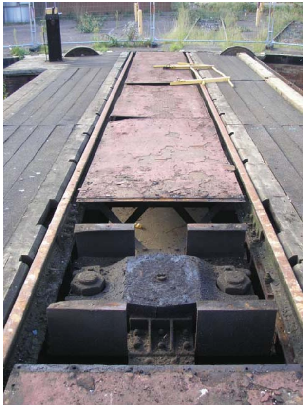
Plate 30. Metal plate removed revealing central turntable pivot.
