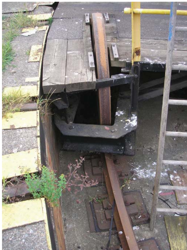
Plate 6. Exposed turntable race wheel, platform edge and track.
