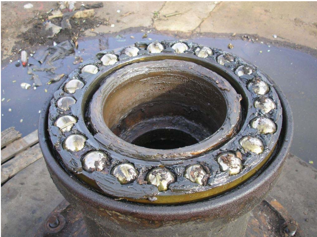
Plate 56. Greased ball bearings on top of central pivot.
