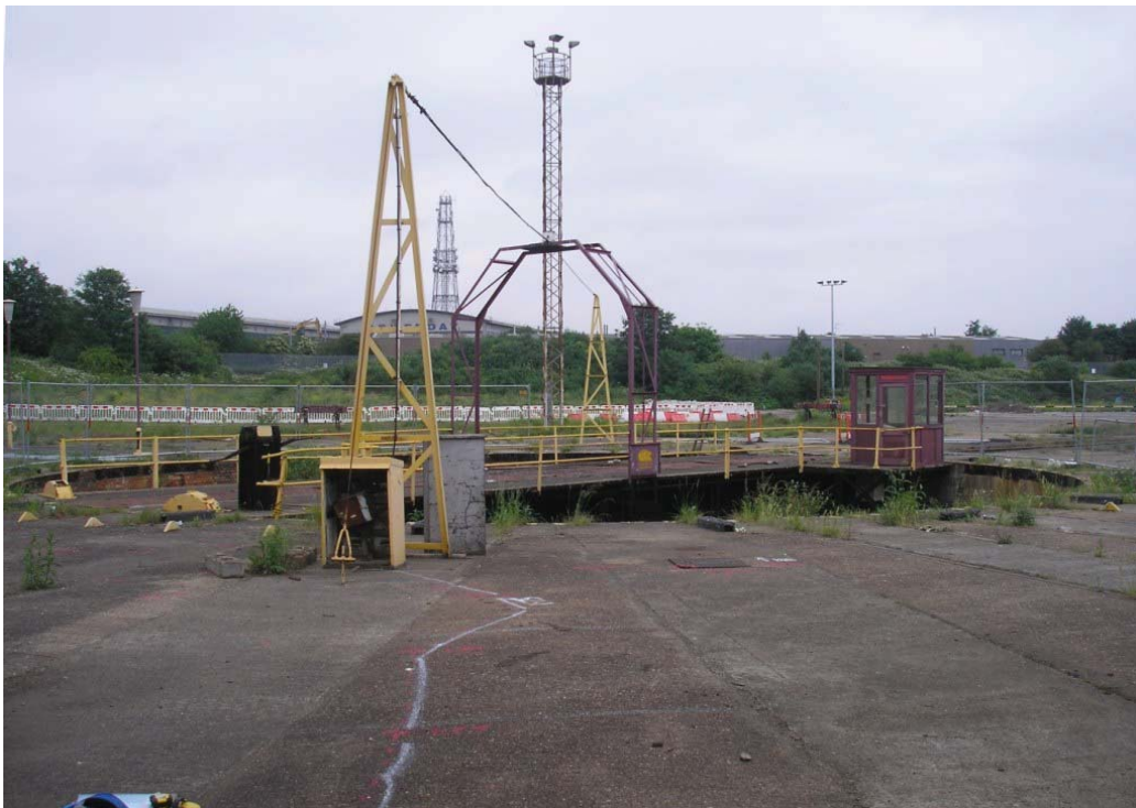
Plate 20. Turntable viewed from the south. The arched 'collector' frame over the turntable was embossed with the makers name 'Cargo Fleet England' and carried a power cable for the electric drive motor.
