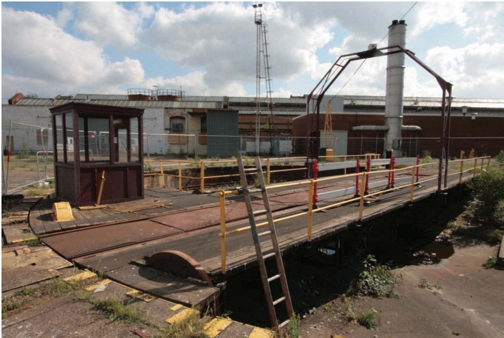
Plate 21. Turntable platform and operator's booth looking south toward Sand Furnace and Pullman Shed Boiler House.
