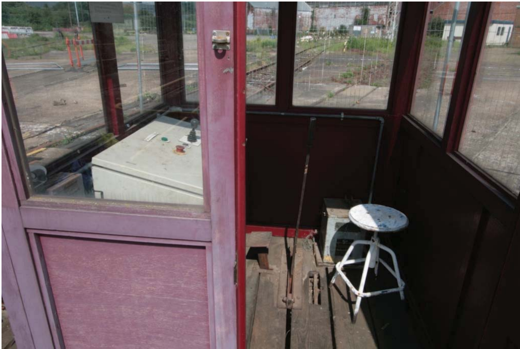
Plate 23. Operator's booth, interior view.
