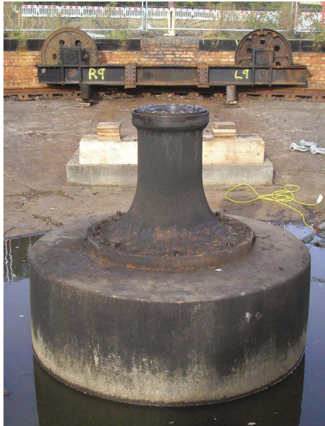
Plate 55. Pivot and 'electric' drive bogie after turntable lifted off.
