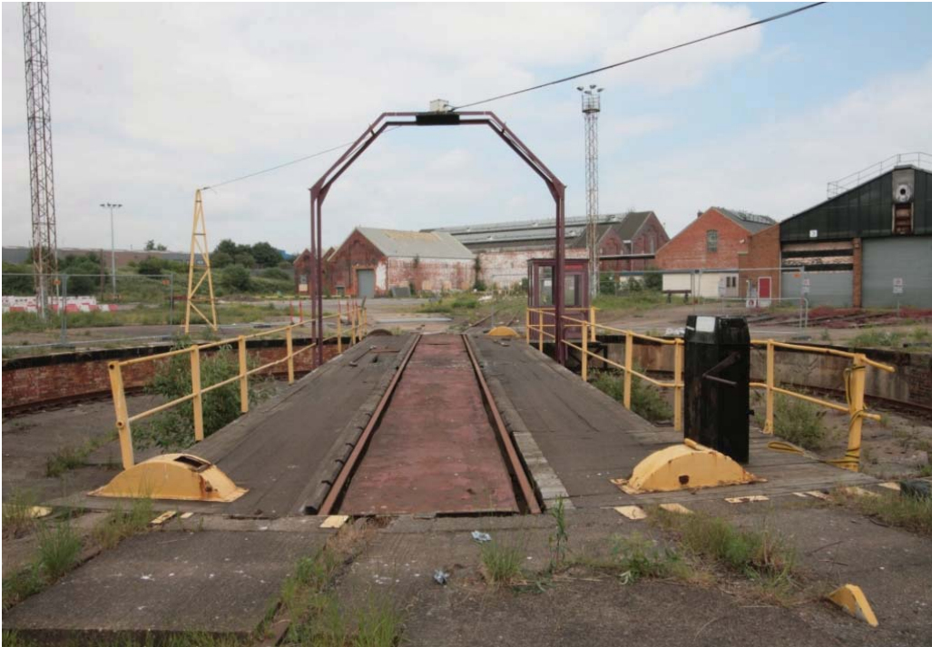
Plate 5. Turntable platform with hand crank mechanism on right and operator's booth at far end. Turntable wheels are beneath the arched metal covers in the foreground.
