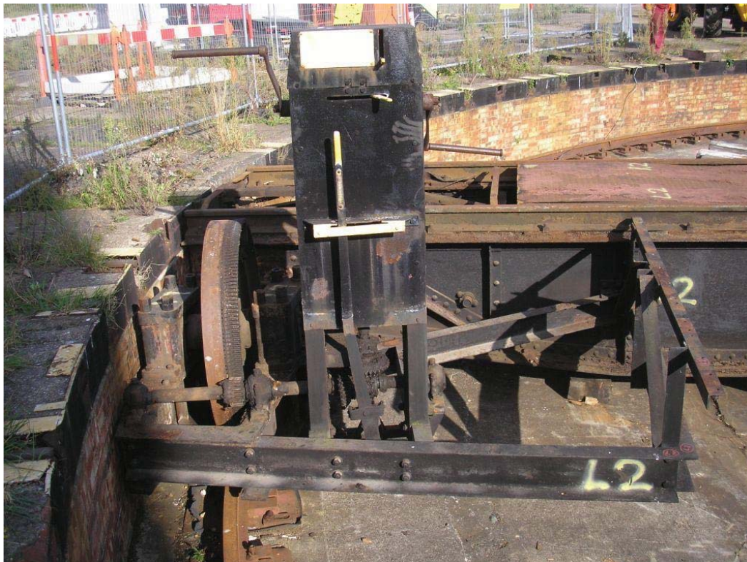
Plate 34. Manual drive mechanism and supporting framework revealed after deck removed.
