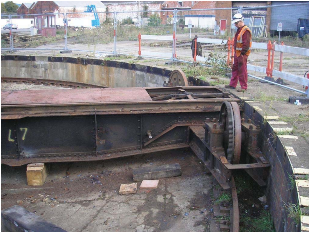
Plate 46. Turntable with electric drive unit removed. The only component that required cutting for the separation was the locking bolt shaft which can be seen in the centre of the turntable side panel.
