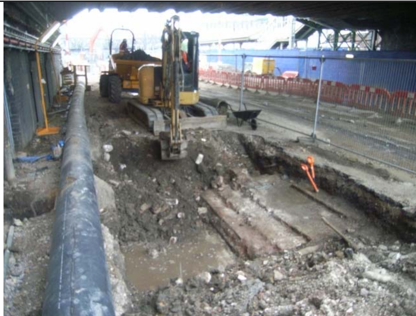
Plate 1: Exposure of northern abutments
