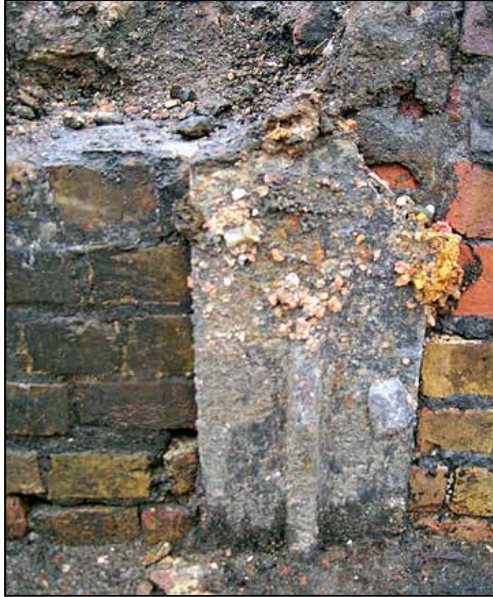
Plate 23: Metal fixtures on pit sidewall [8746]
