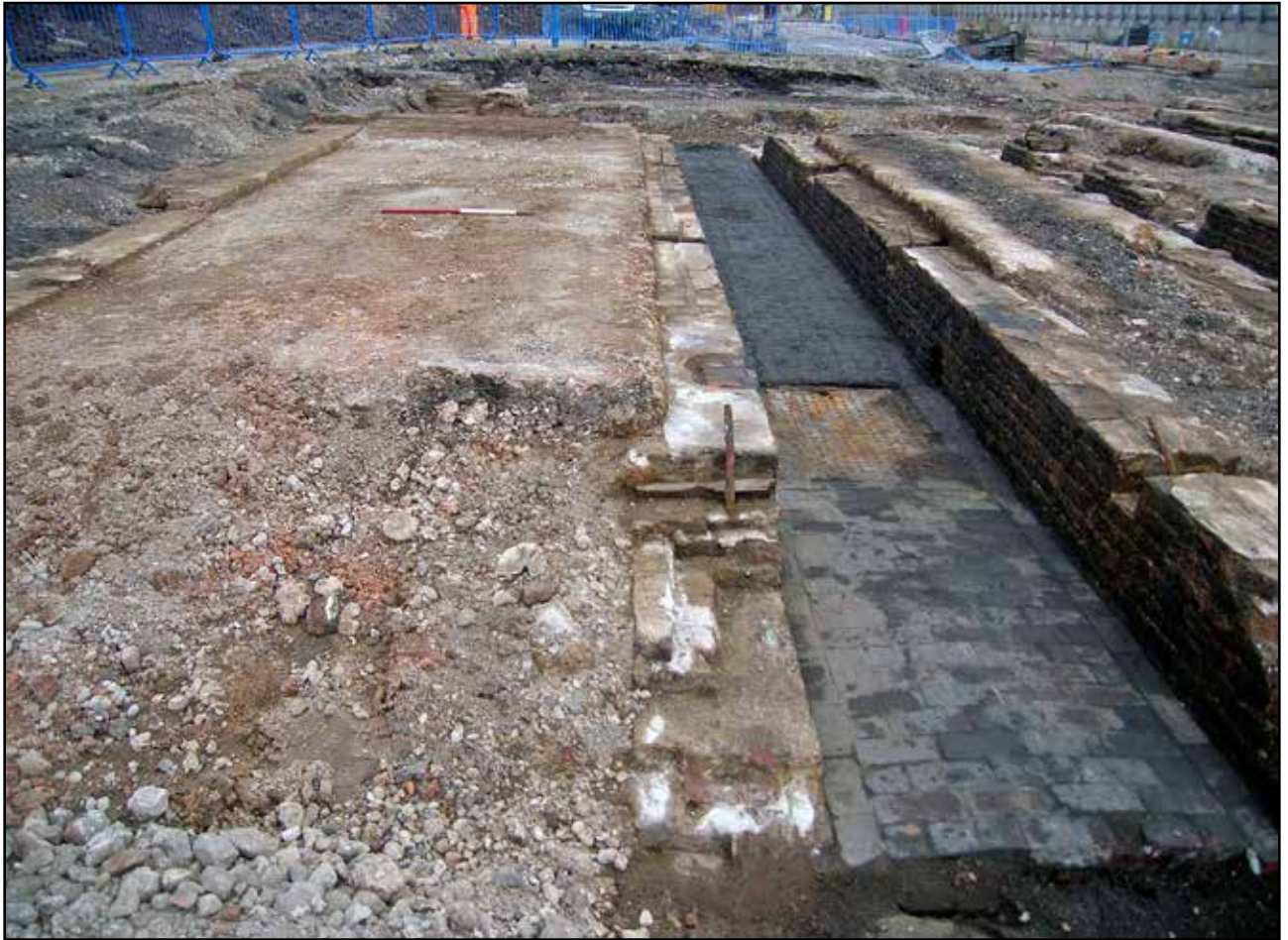
Plate 13: Western end of 1861 inspection pit showing catchment pit [8685] and sleeper cuts. The floor of shed (8681) is to the left
