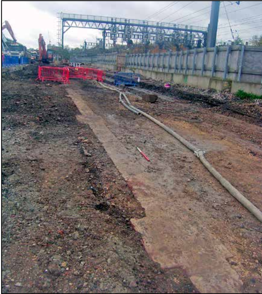
Plate 47: Northern wall of Broad gauge shed
