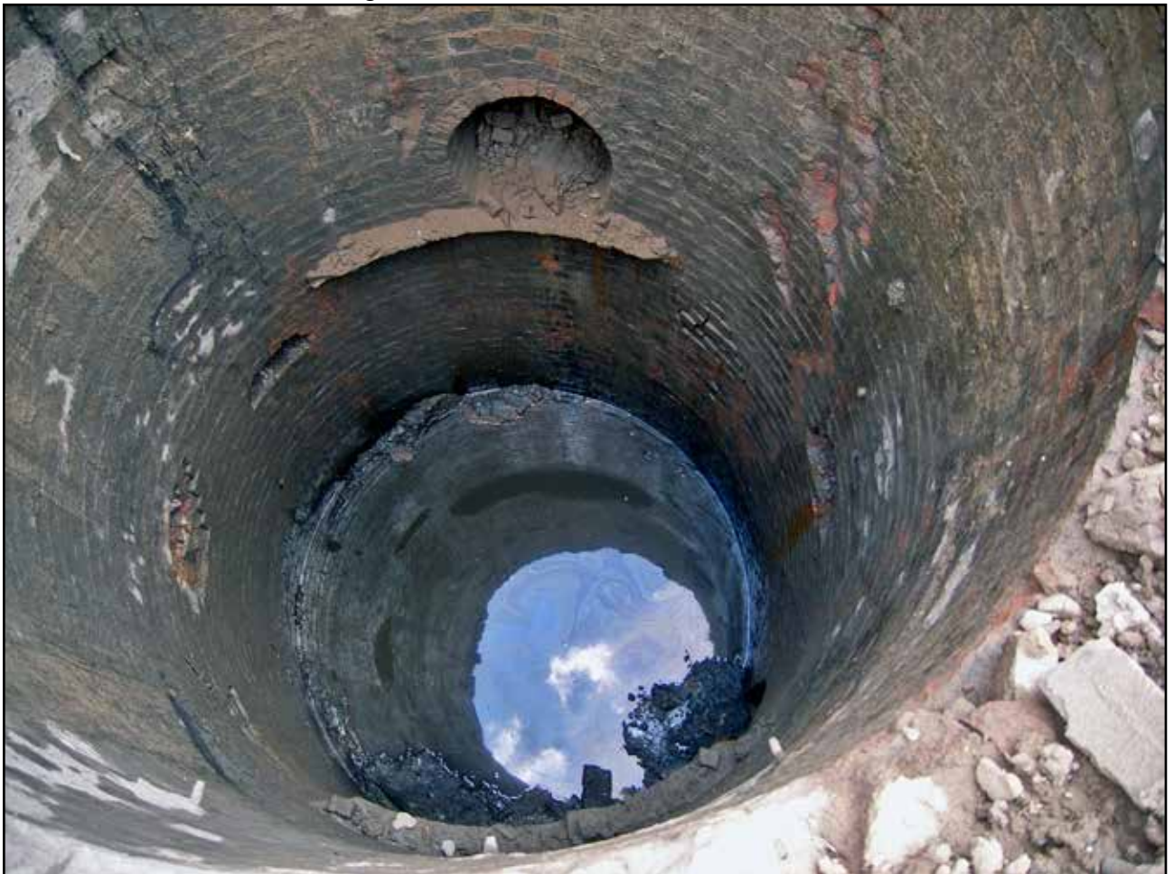
Plate 44: Base of [8227] showing entrance to [8251] and [8250]
