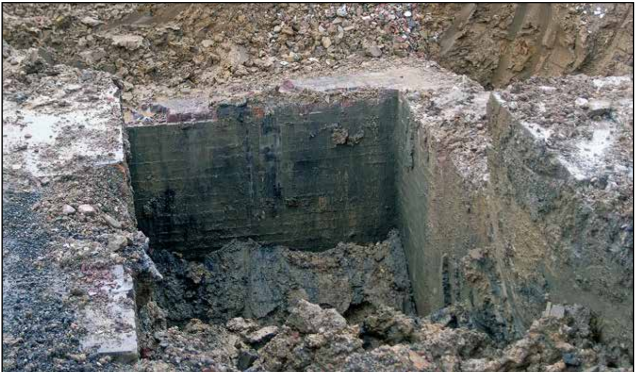
Plate 16: Brick Tank [8828] to north of 1861 shed
