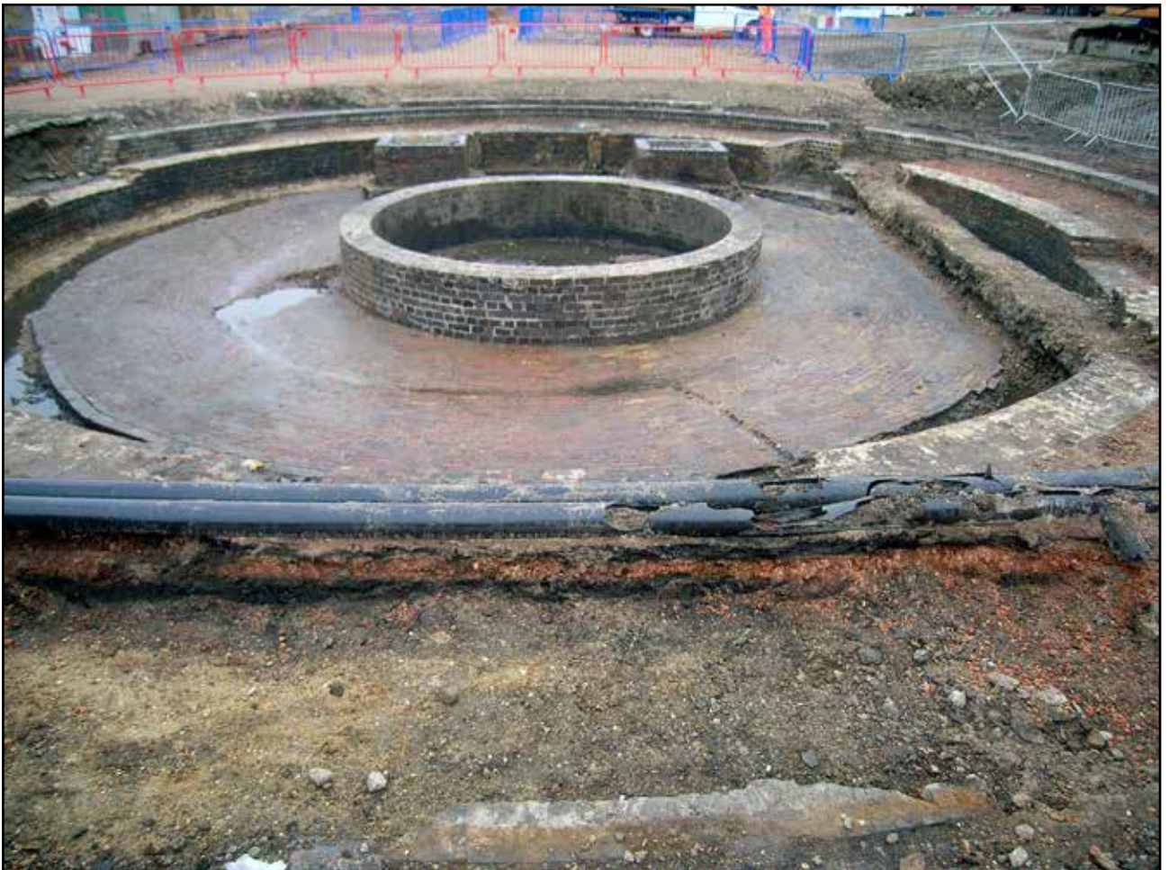
Plate 22: Turntable pit from east
