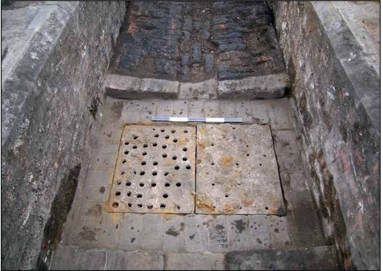
Plate 49: Catchment pit [8358] in base of inspection pit
