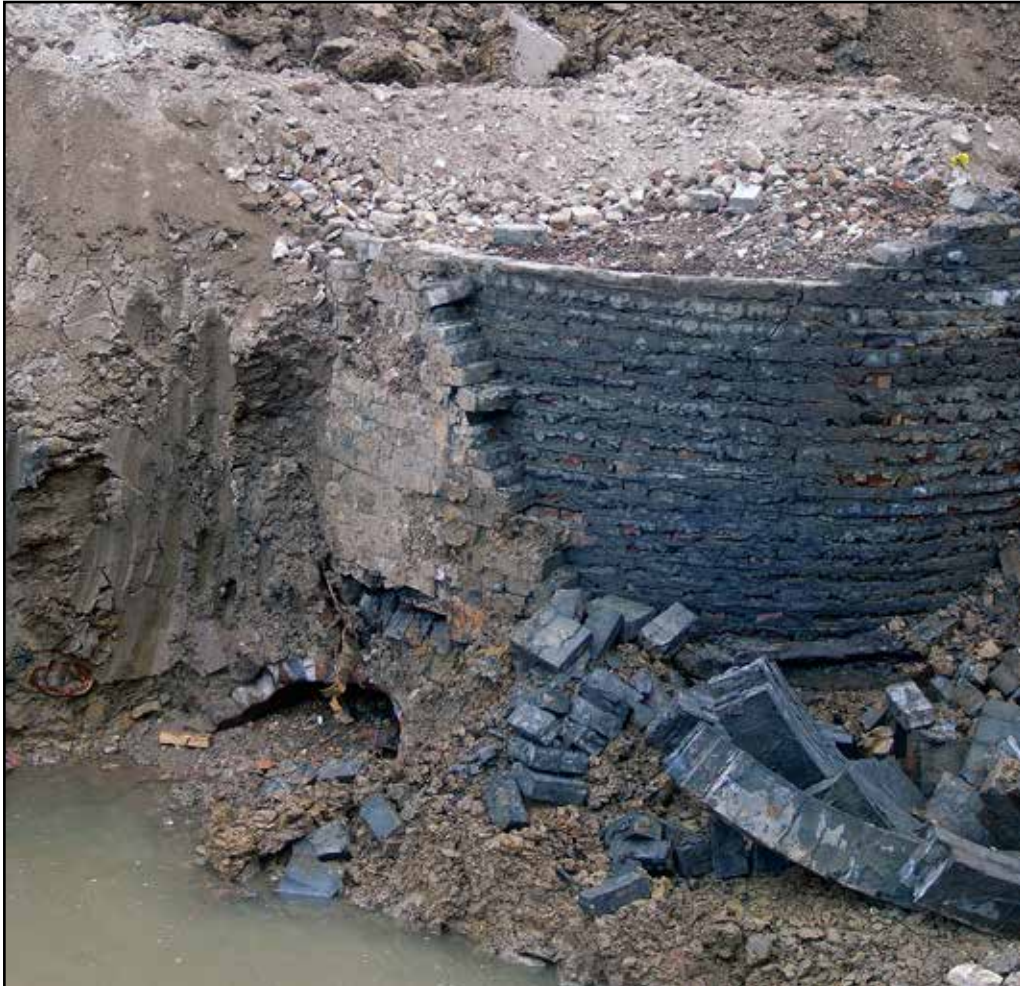
Plate 43: Shaft 8206 showing double skinned wall
