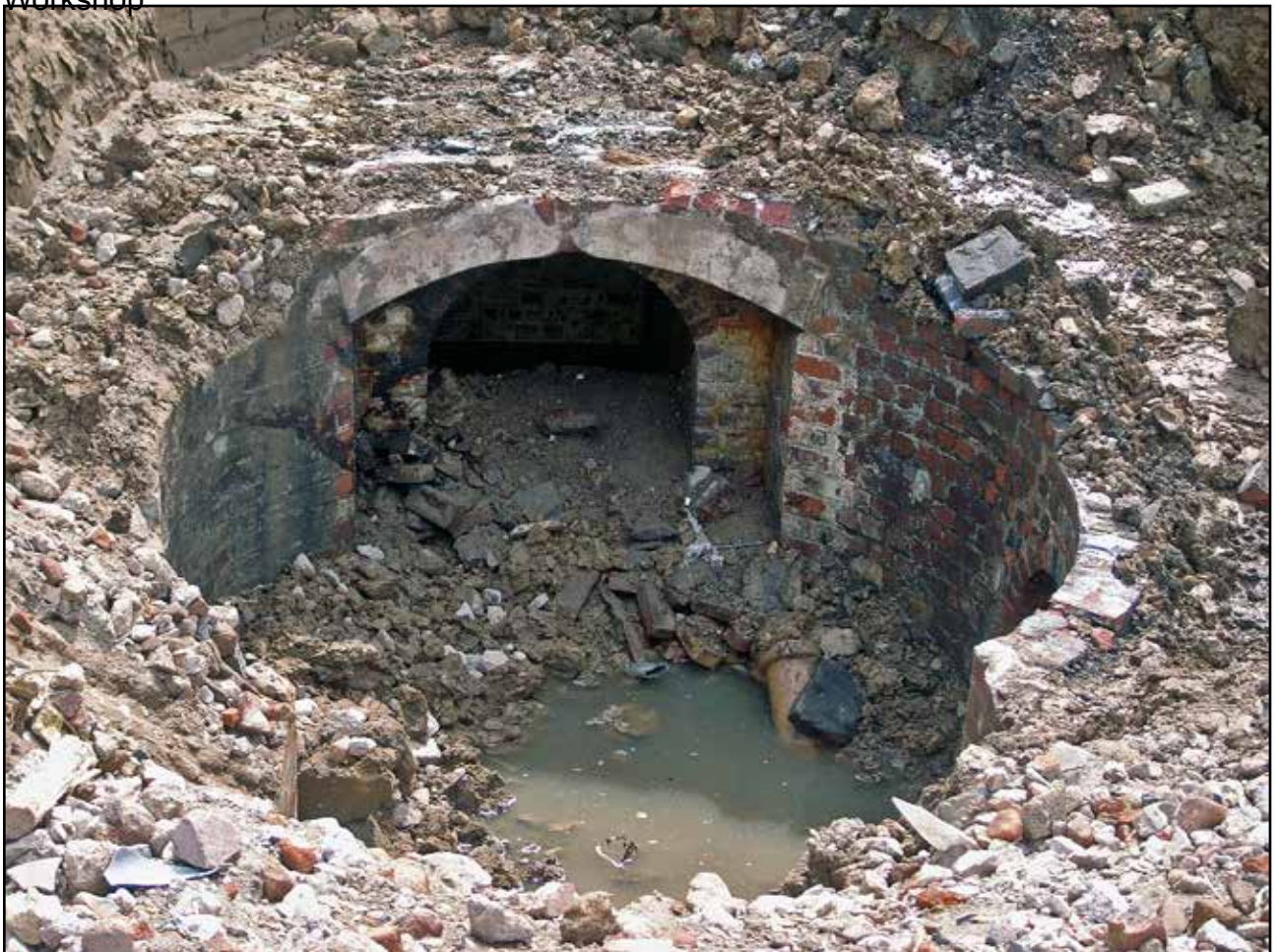
Plate 40: Upper level 8201 of shaft [8236] showing room [8211] and entrance to conduit [8213]
