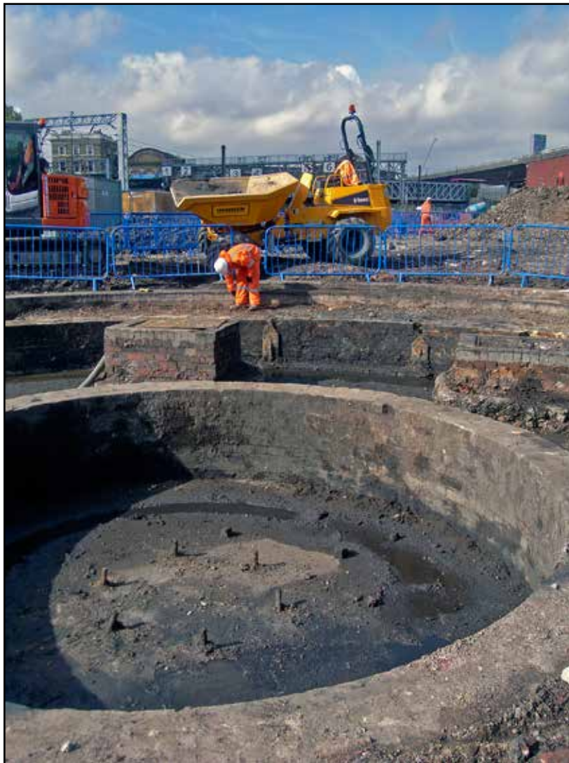
Plate 24: Centre of Turntable pit showing phase 2 wall [8747]
