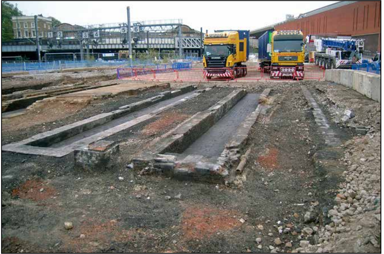
Plate 19: Inspection pits [8786] and [8785] of 1871 shed from east
