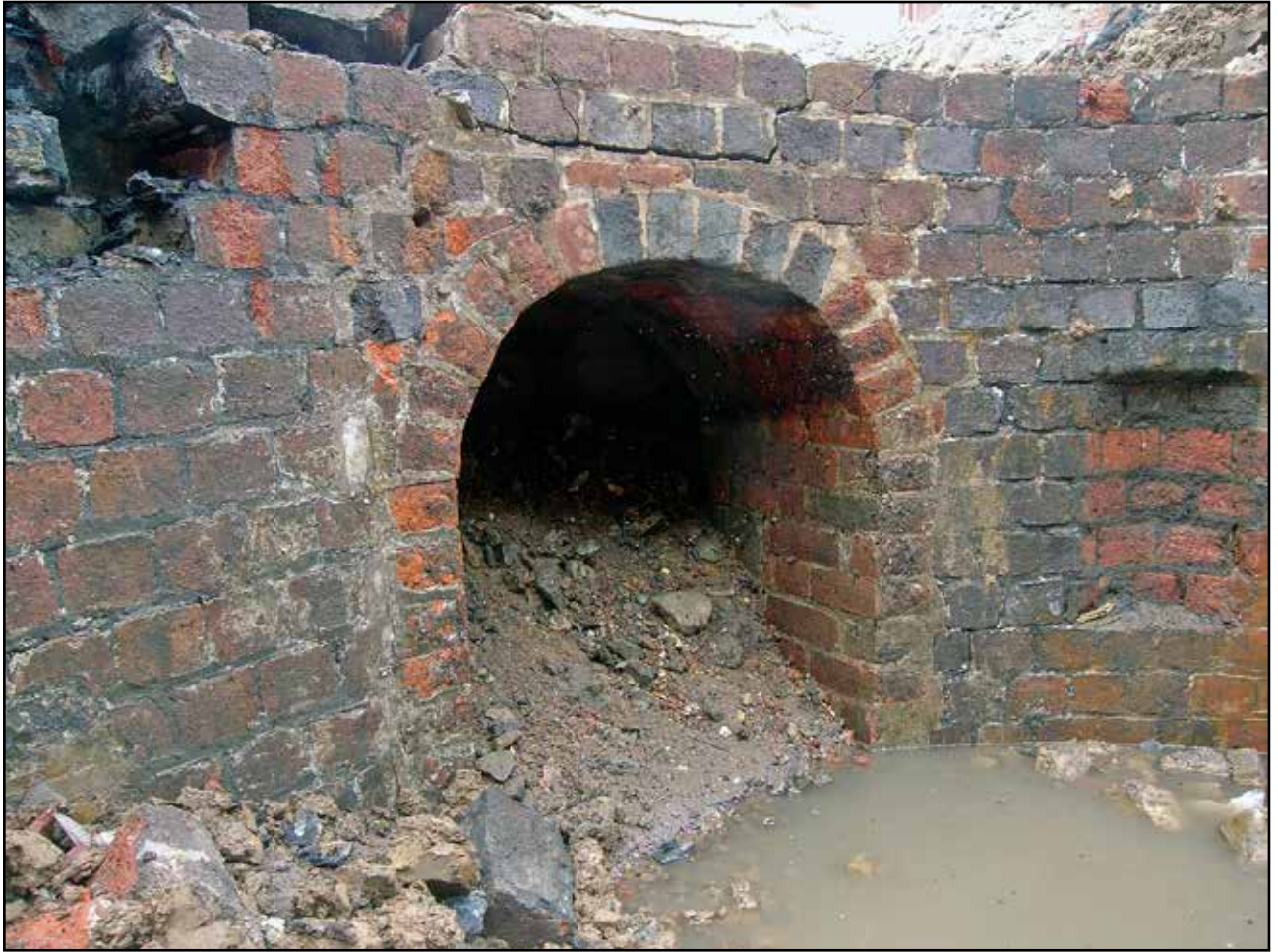
Plate 41: Base of upper level [8201] showing arched entrance to conduit [8213]
