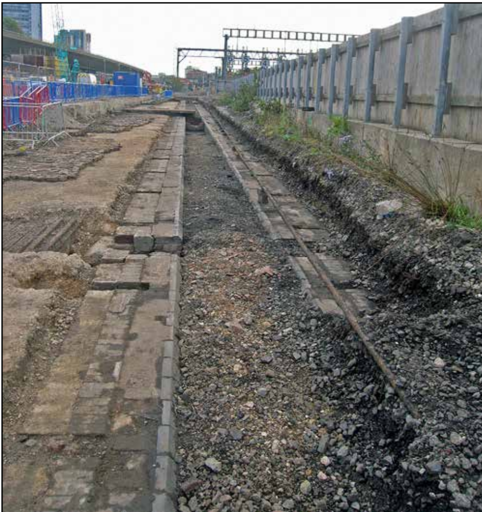
Plate 50: Partly excavated inspection pit
