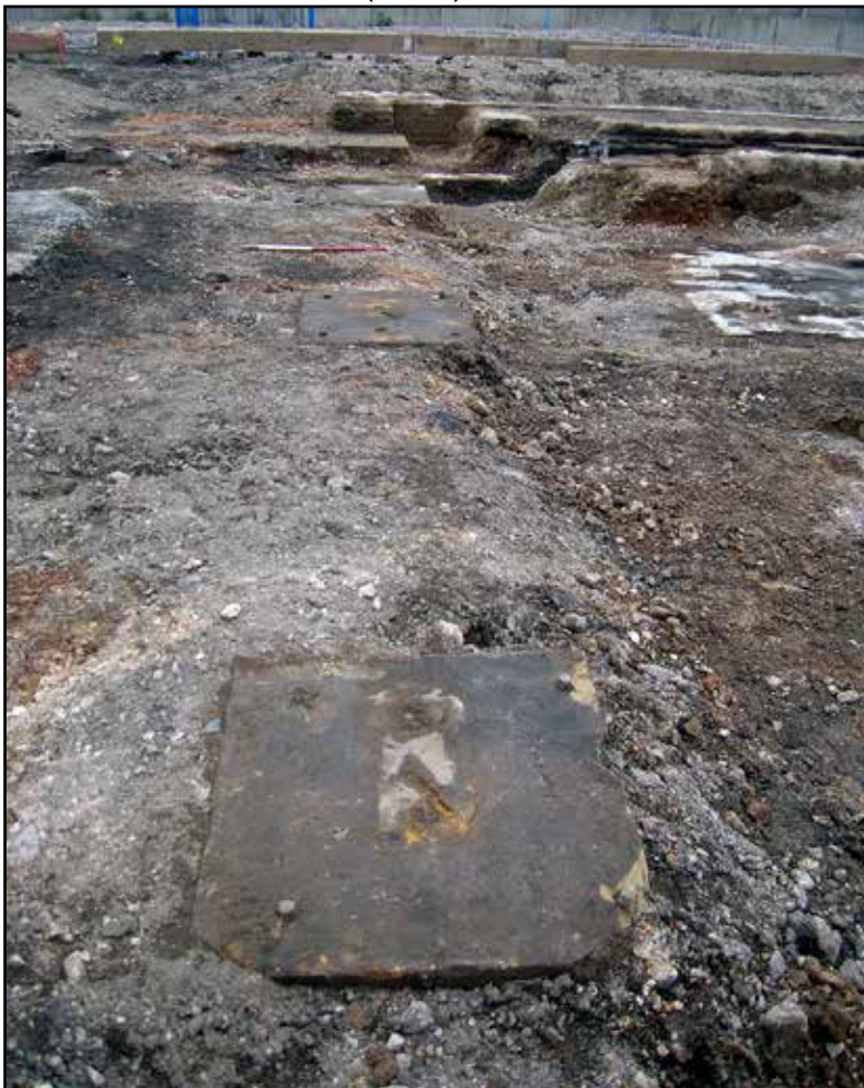
Plate 14: Eastern end of 1861 shed showing row of stone plinths for metal columns
