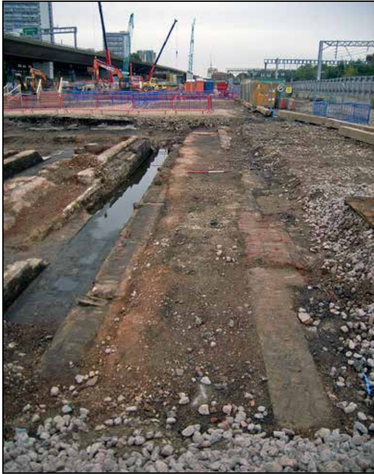
Plate 11: Southern outer wall [8699] of 1861 shed
