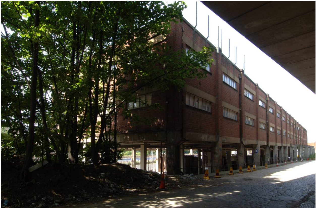
Fig 15 the north elevation of the building looking west
