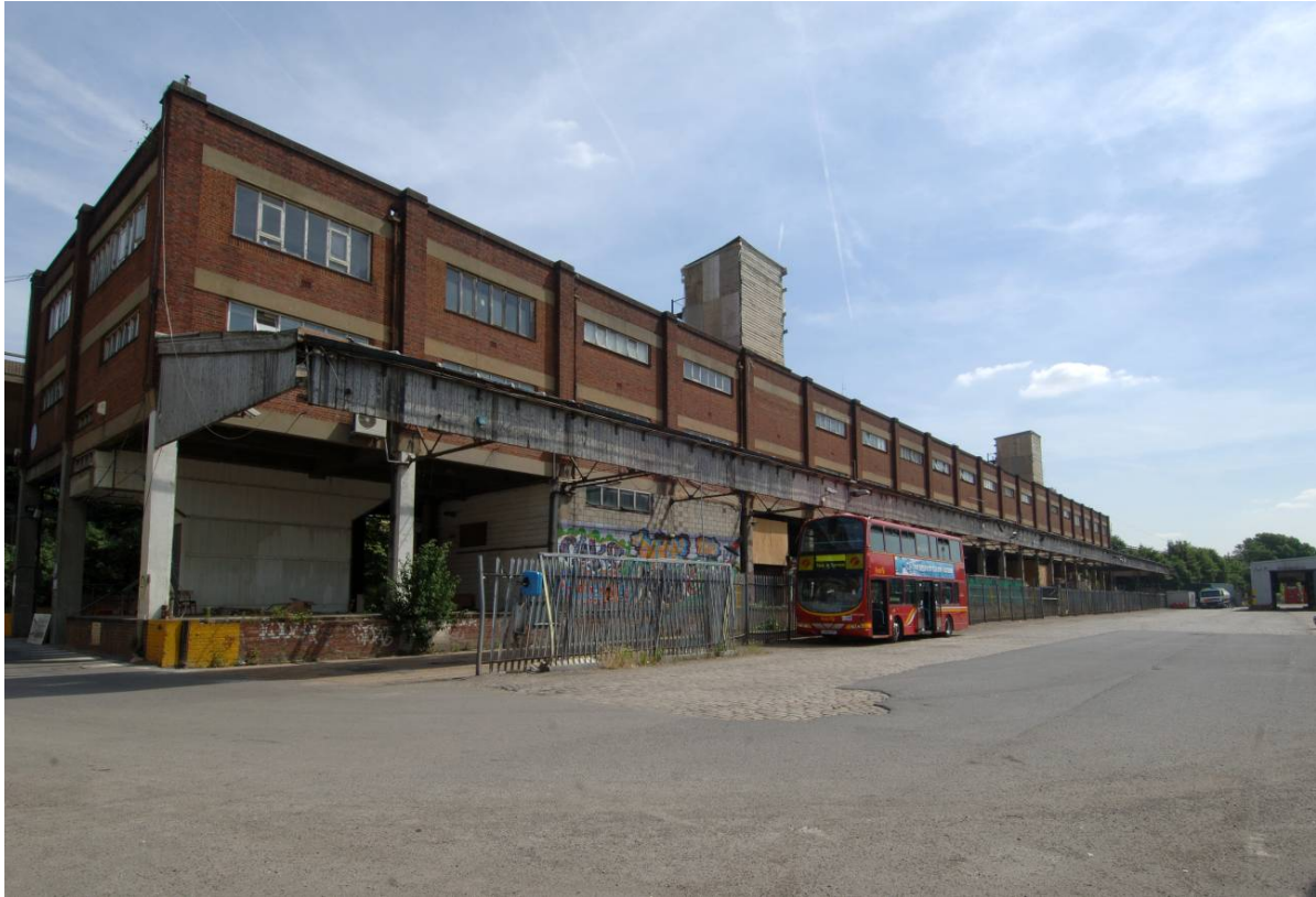
Fig 5 the Great Western Studios or former goods yard building, looking north-east
