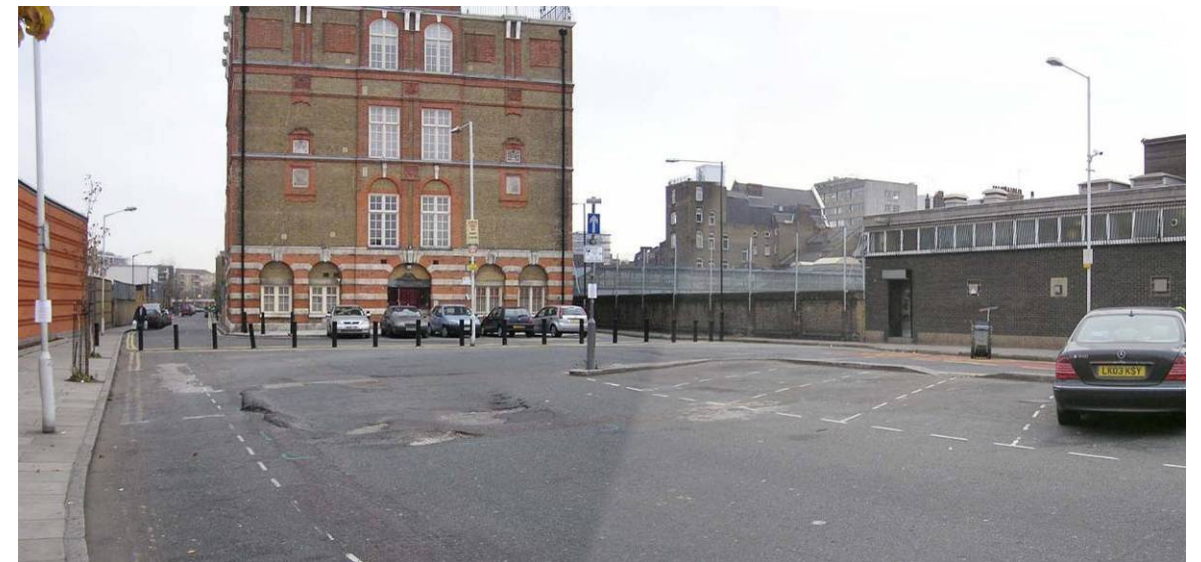
Figure 12-6-Durward Street – worksite area for Fulbourne Street Ticket Works
