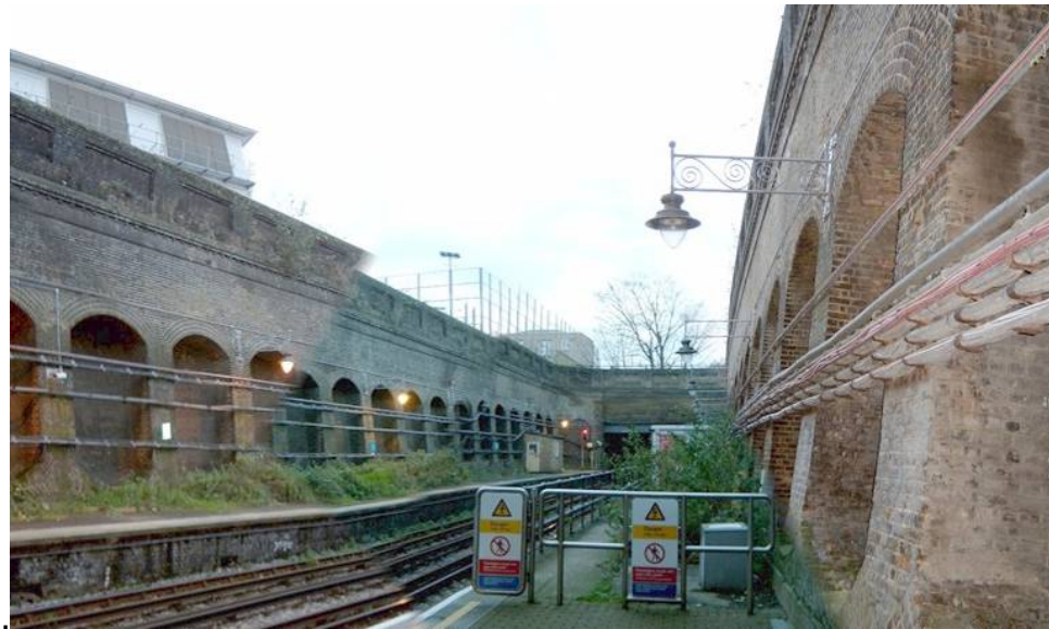
Figure 12-1-ELL Cutting at Intermediate Concourse Location
