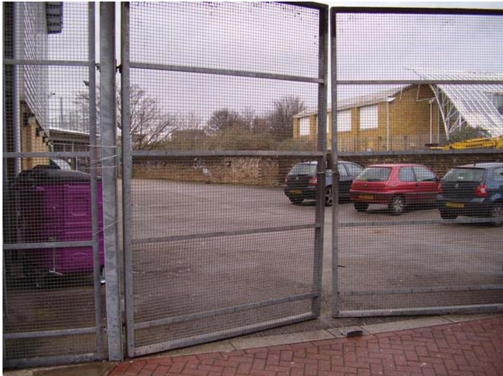
Figure 5. Part of the Durward Street Shaft and Interchange site visible from Durward Street
