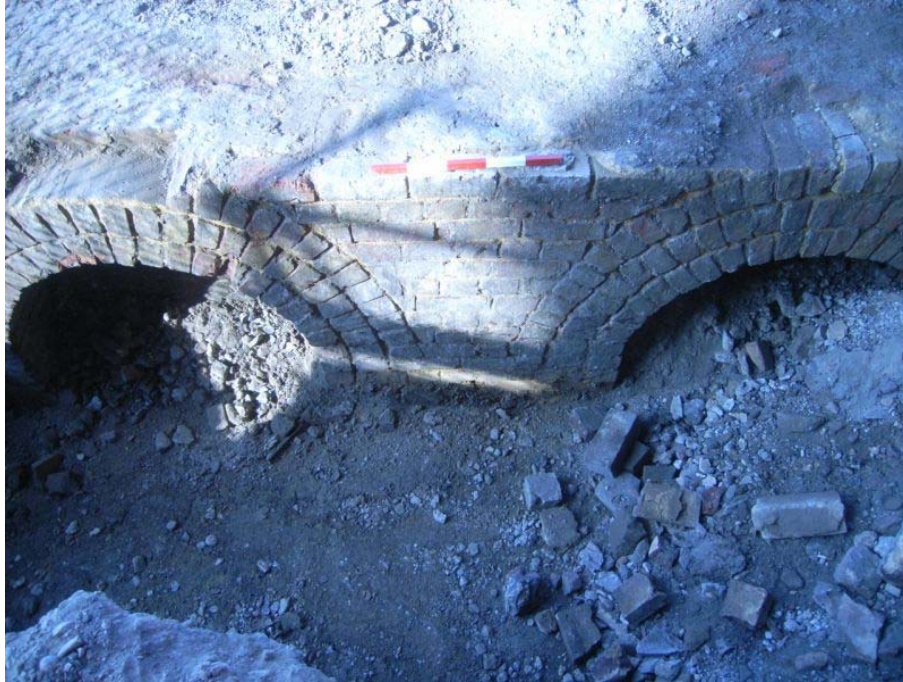
Plate 16: Room 5 - the arched recesses in wall 7088, looking south-west
