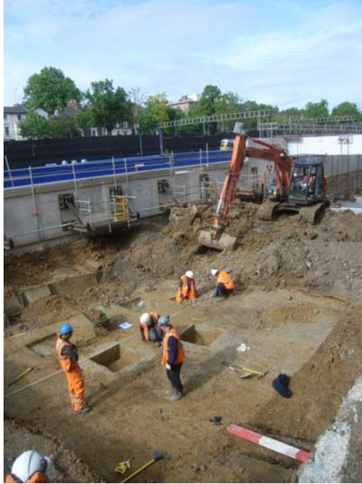
Plate 6: Manual test pitting through the lower brickearth deposits, the channel deposits and the colluvial gravels, looking south-west
