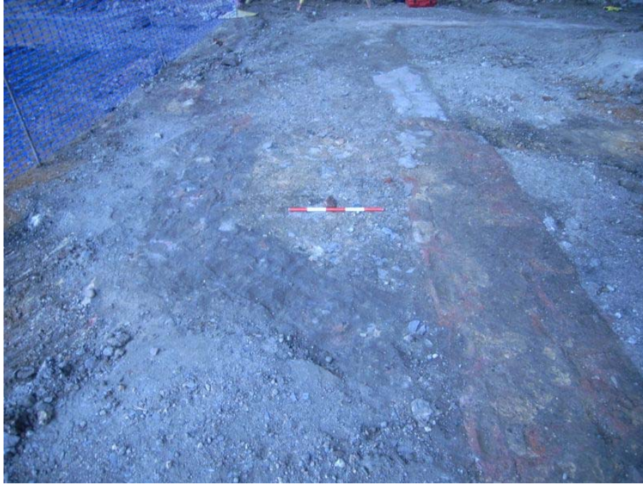
Plate 20: Additional brick bay structure 7090, abutting wall 7093, with wall 7096 in the distance. Looking north-west
