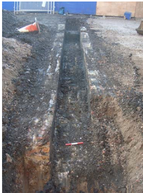
Plate 7: Service/Utilities channel (2051) from north
