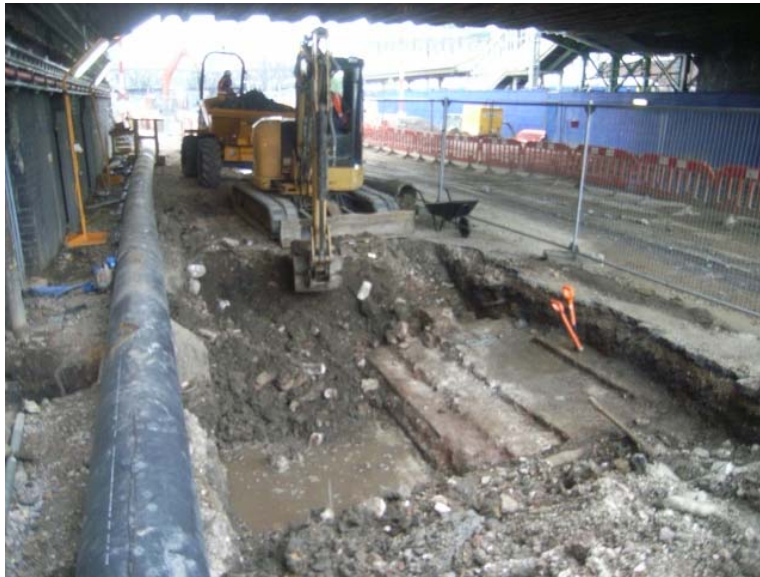
Plate 1: Exposure of northern abutments
