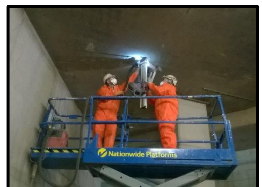
Mounted drilling rig
