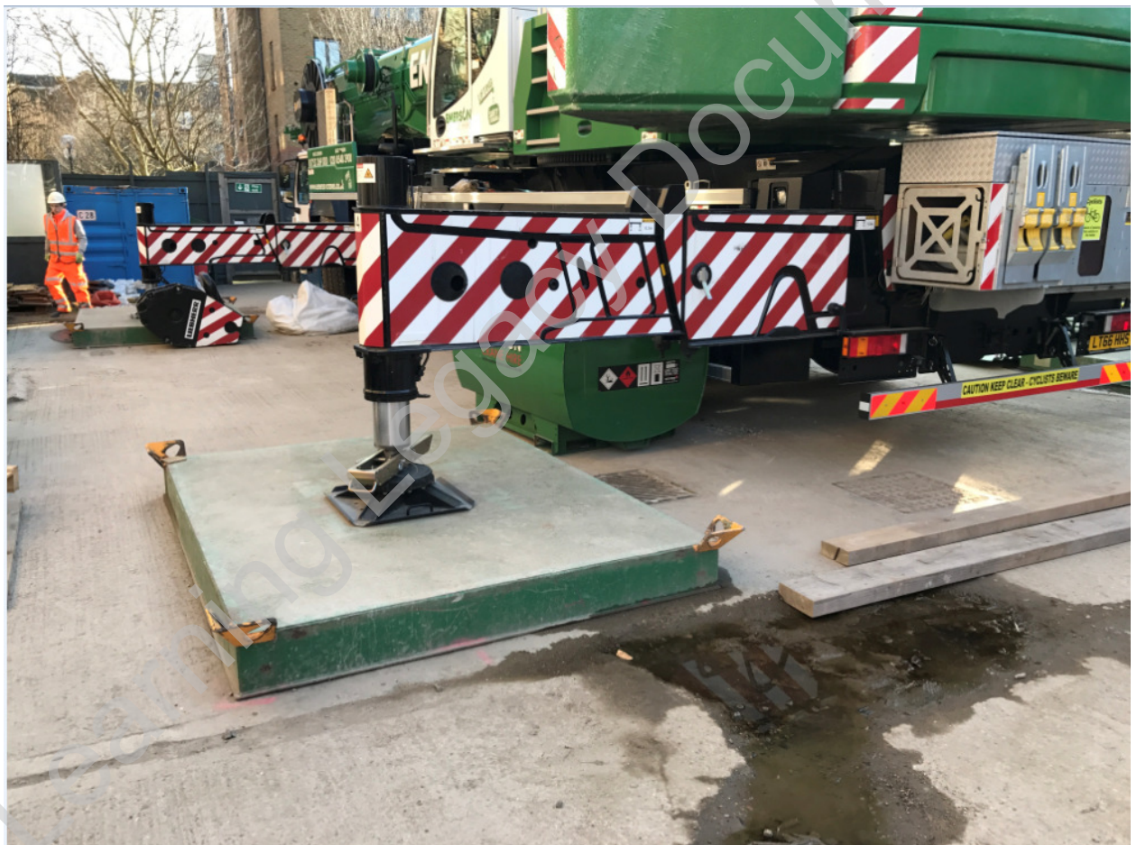
Figure 7 -C512 Site Obstruction resurface concrete slab
